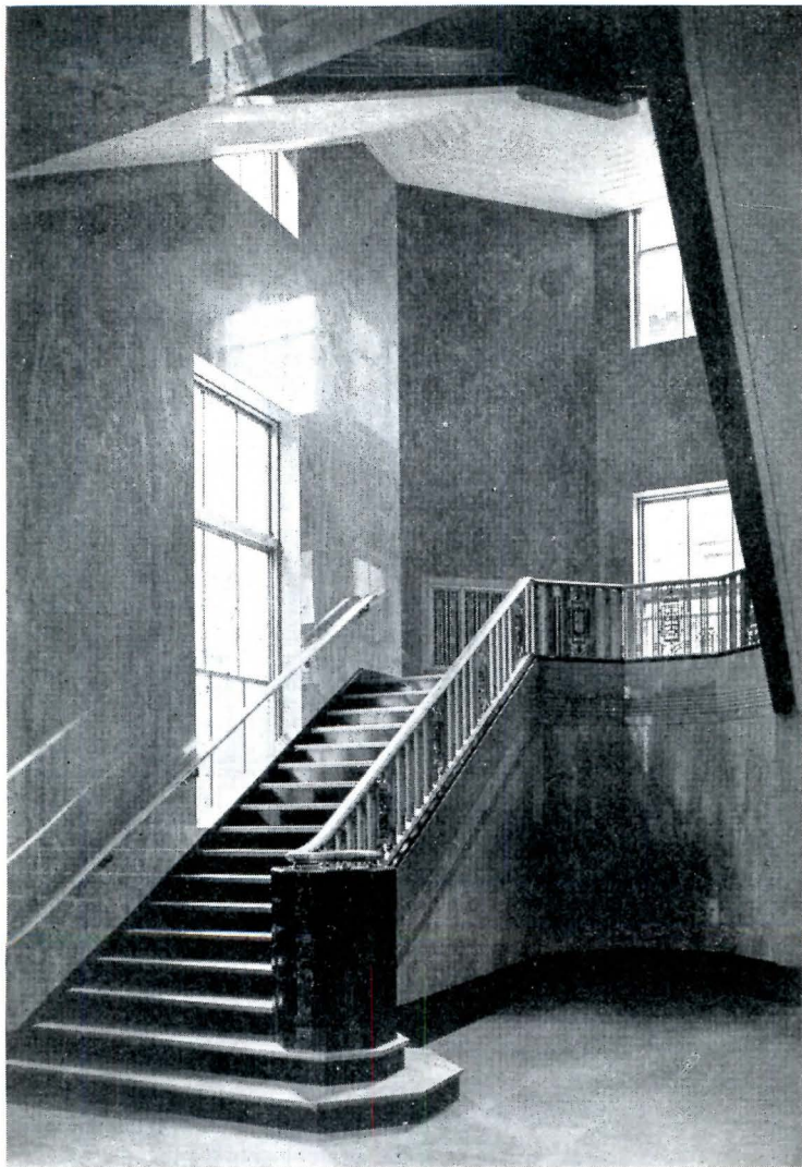
ONE OF TWO MAIN STAIRWAYS, NEW ALBANY POST OFFICE, ALBANY, N. Y.
