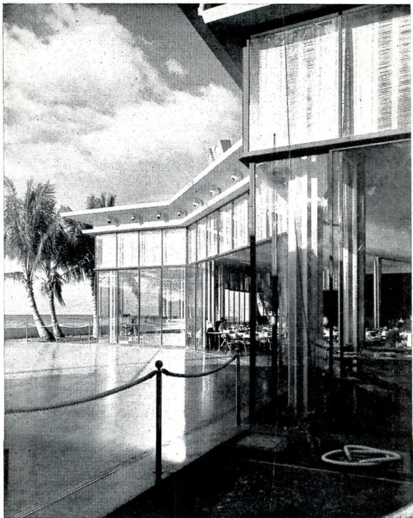
OUTDOOR DINING-ROOM AN ADDITION TO THE ROYAL HAWAIIAN HOTEL, HONOLULU GARDNER A. DAILEY, ARCHITECT
