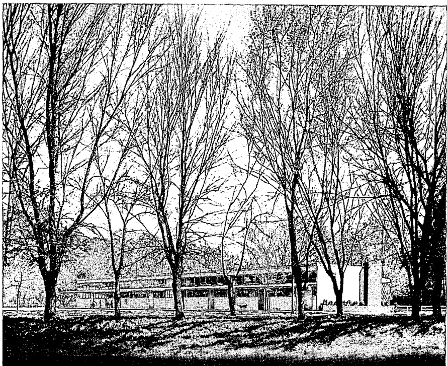
ATASCADERO ELEMENTARY SCHOOL, ATASCADERO, CALIF. DANIEL, MANN & JOHNSON, ARCHITECTS .
