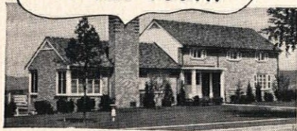
Residence of W. Marshall Hughes, A.I.A., Wyomissing Hills, Reading, Pa. Architect: W. Marshall Hughes. Builder: W. M. Hughes & Son, Inc. Heating Contractor: Corbit's, Inc.
