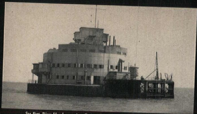
Sea Fort, River Humbee; an installation of Hope's Hot-Dip Galvanized Windows
