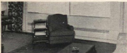
Living room in typical apartment showing Webster Walvector.
