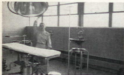
Operating Room. Webster Walvector offsets heat loss from large glass exposures here and in nursery and obstetric suite.
