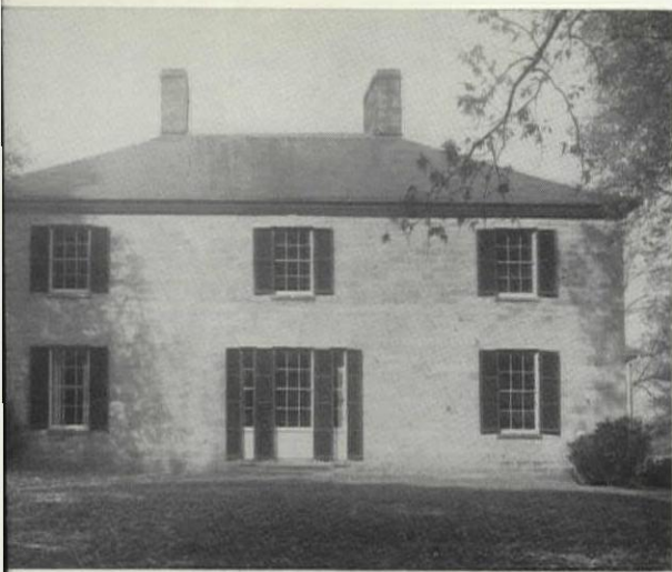
LEFT PHOTOGRAPH OF A STEREOPAIR OF THE SOUTH FACADE OF ADENA.
