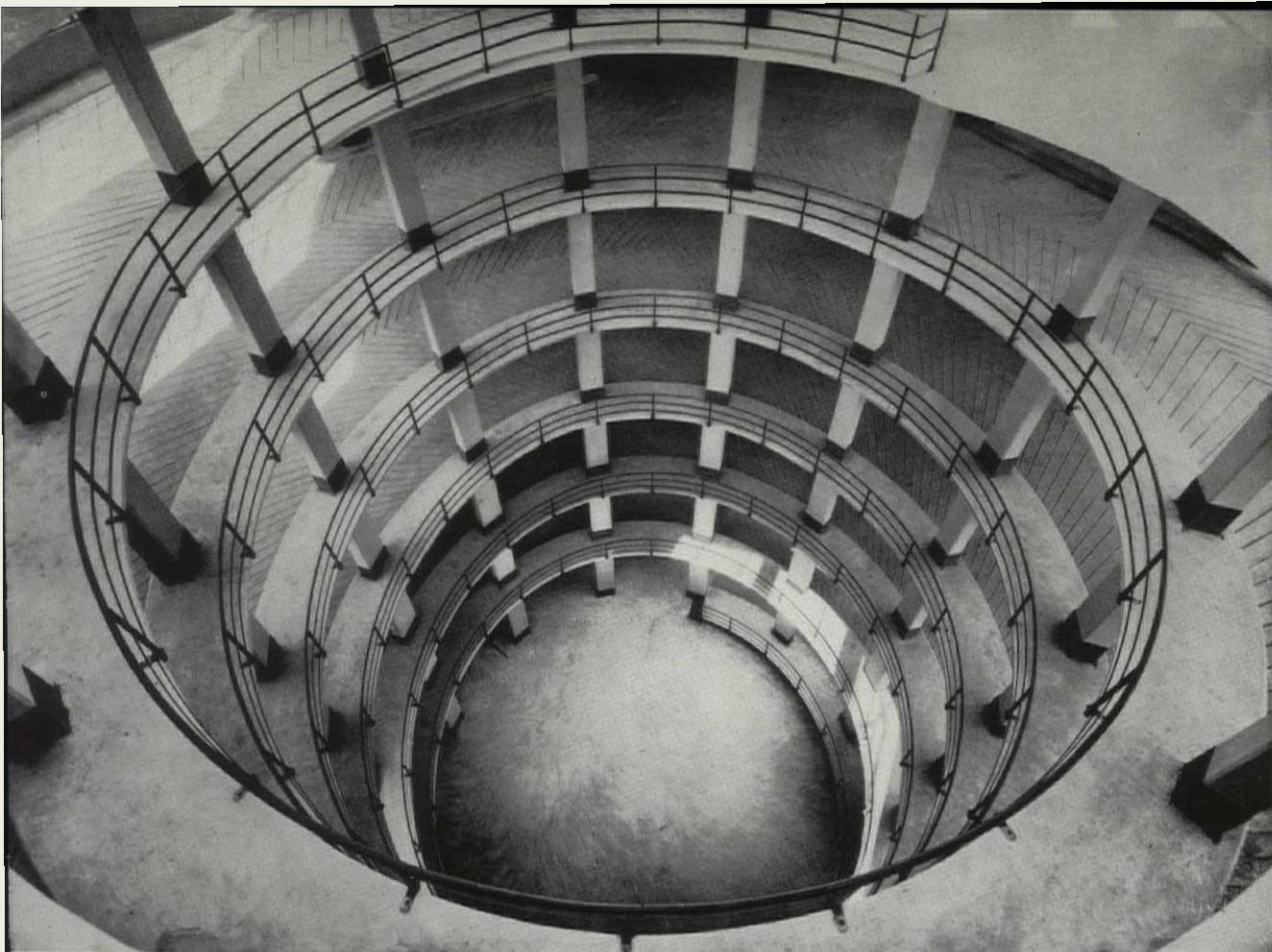
CIRCULAR RAMP — VENICE, ITALY
