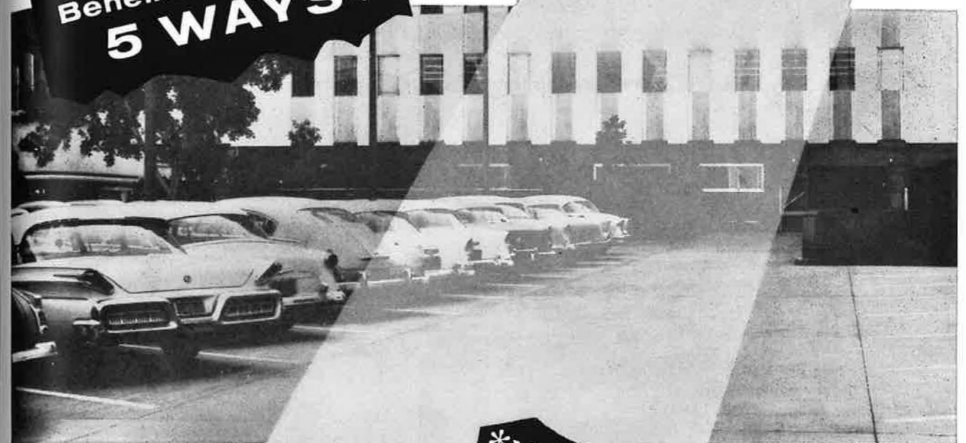
550 South Flower Bldg. Los Angeles, Calif. Claud Beelman, Architect Robert E. Bauman Co. (Concrete Sealing)
