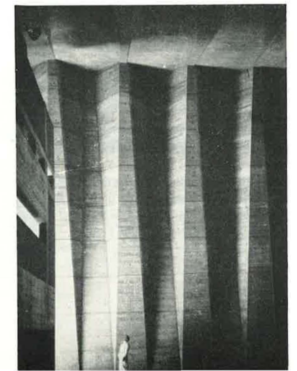
Unesco House, Paris. Interior of Conference Hall.
