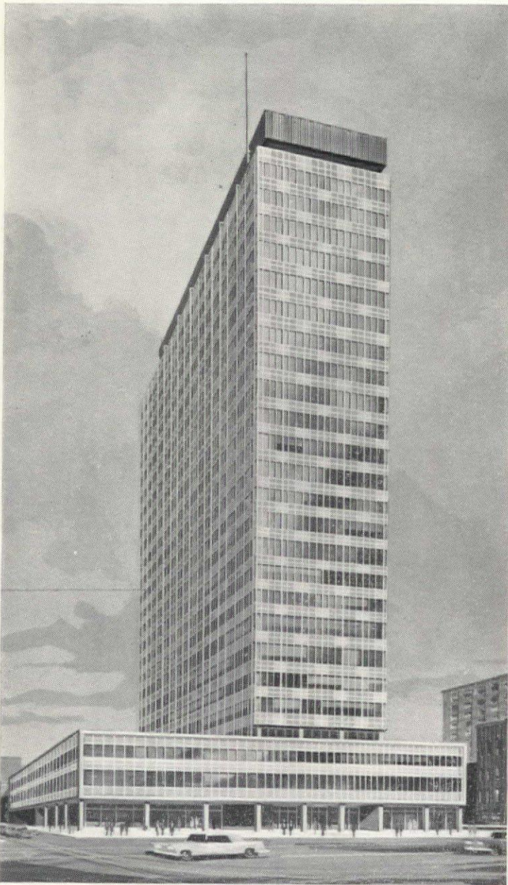
KROGER BUILDING, Cincinnati, Ohio. Owner: R. E. Dumas Milner. Architects and Engineers: Hedrick and Stanley, Fort Worth, Texas. Plumbing Contractor: Sam P. Wallace & Company, Cincinnati, Ohio.
