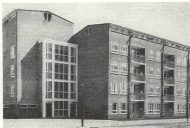
Amsterdam-West. Middle income housing, with access galleries on one side and private balconies on the other.
