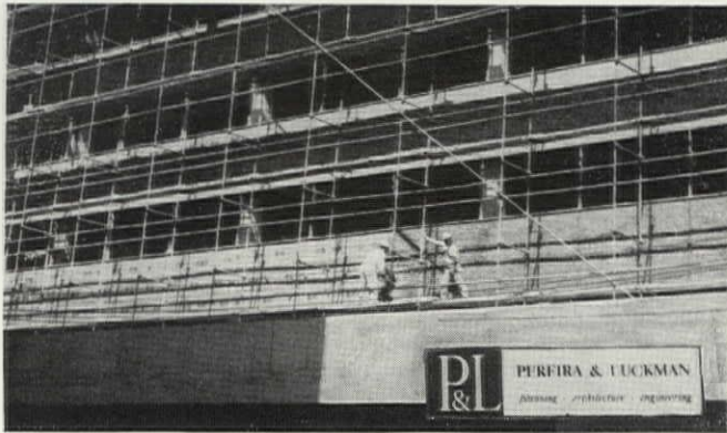
The 13-story Los Angeles IBM office building with K-LATH spandrel walls. Pereira & Luckman, architects.
