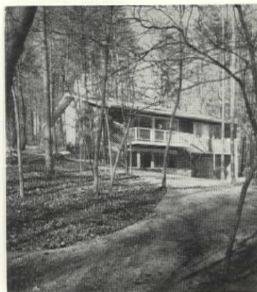
Flint Hill, Bethesda, Maryland. Forty-five houses on half-acre lots, $32,000 to $38,000. Bennett Construction Company, 1958-59
