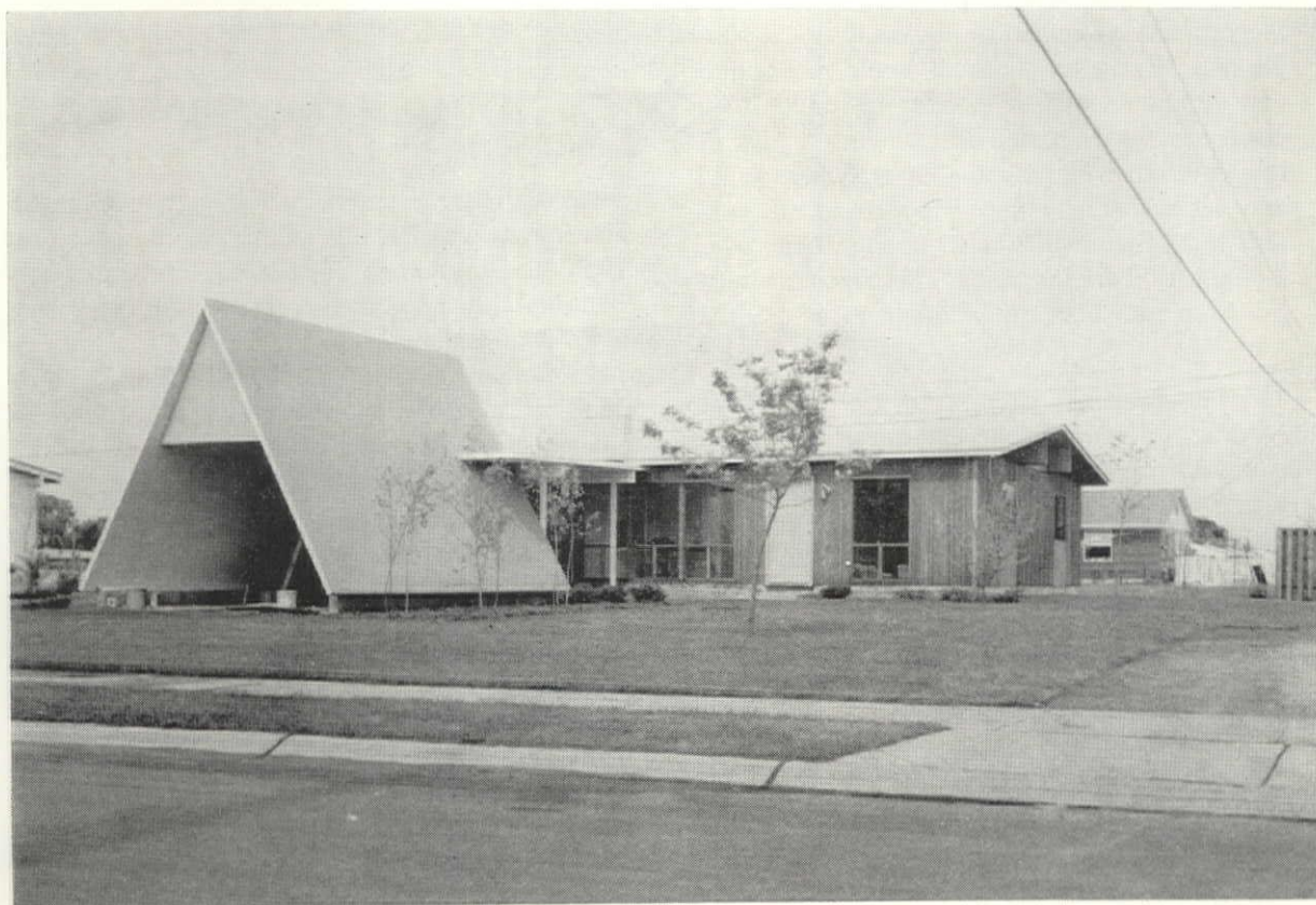
The Research House for 1958 at South Bend, Indiana, designed by the Research Institute of the National Association of Home Builders with Herman York as Consulting Architect. This home utilizes structural insulating panels with interior and exterior finishes molded to a core of Dylite expandable polystyrene foam
