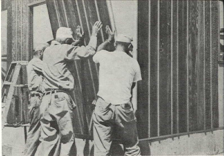
Stressed-skin wall panel placement
