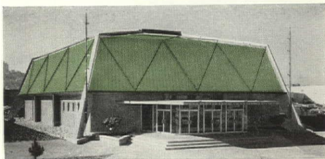
Memorial Building of the International Longshoremen's and Warehousemen's Union, San Francisco. ARCHITECT: Henry Hill, San Francisco. The dome is sheathed with about 18,000 sq. ft. of Economy Copper Roofing installed by Fire Protection Products Co., San Francisco.
