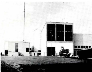
Experimental power-producing reactor
