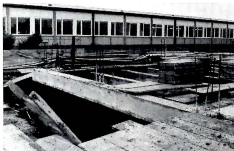
Below, Allgemeine Elektricitats-Gesellschaft (AGE) Electronics Lab, Frankfurt. Left, precast floorslabs can be removed and footings provided for heavy apparatus or utilities brought in. Right, Standard one-story form
