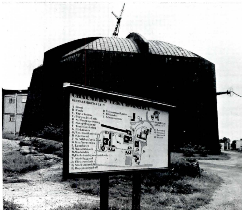
Chalmers Institute of Technology, Gothenburg, Sweden. High tension laboratory, Klas Anselm, architect
