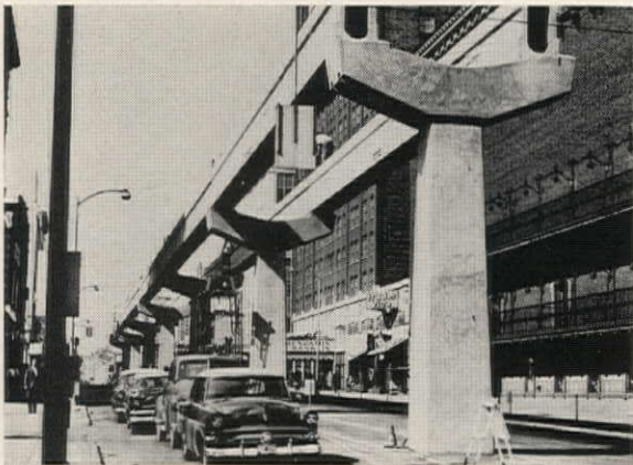
Supporting concrete columns of the Alweg monorail
