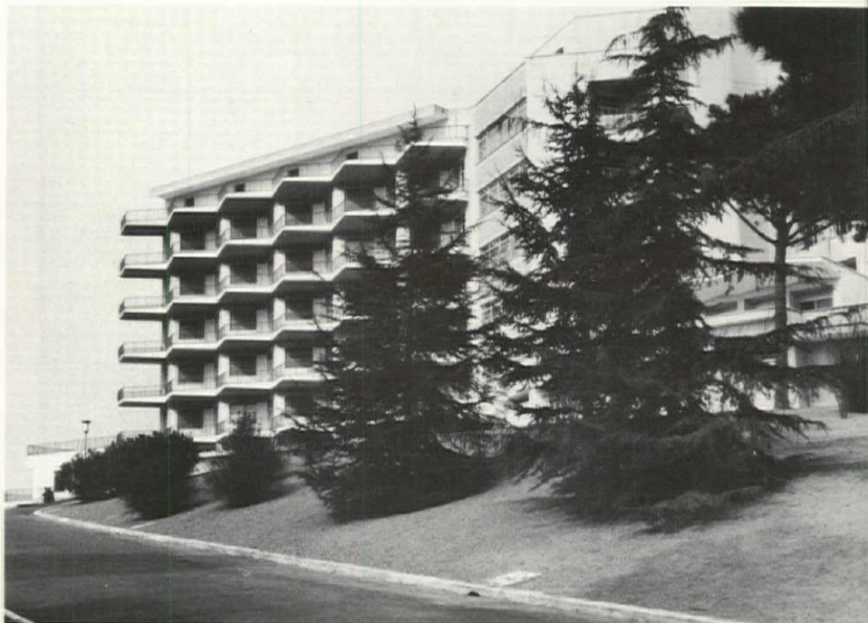
New Traumatology Hospital and Rehabilitation Center, Rome, Italy
