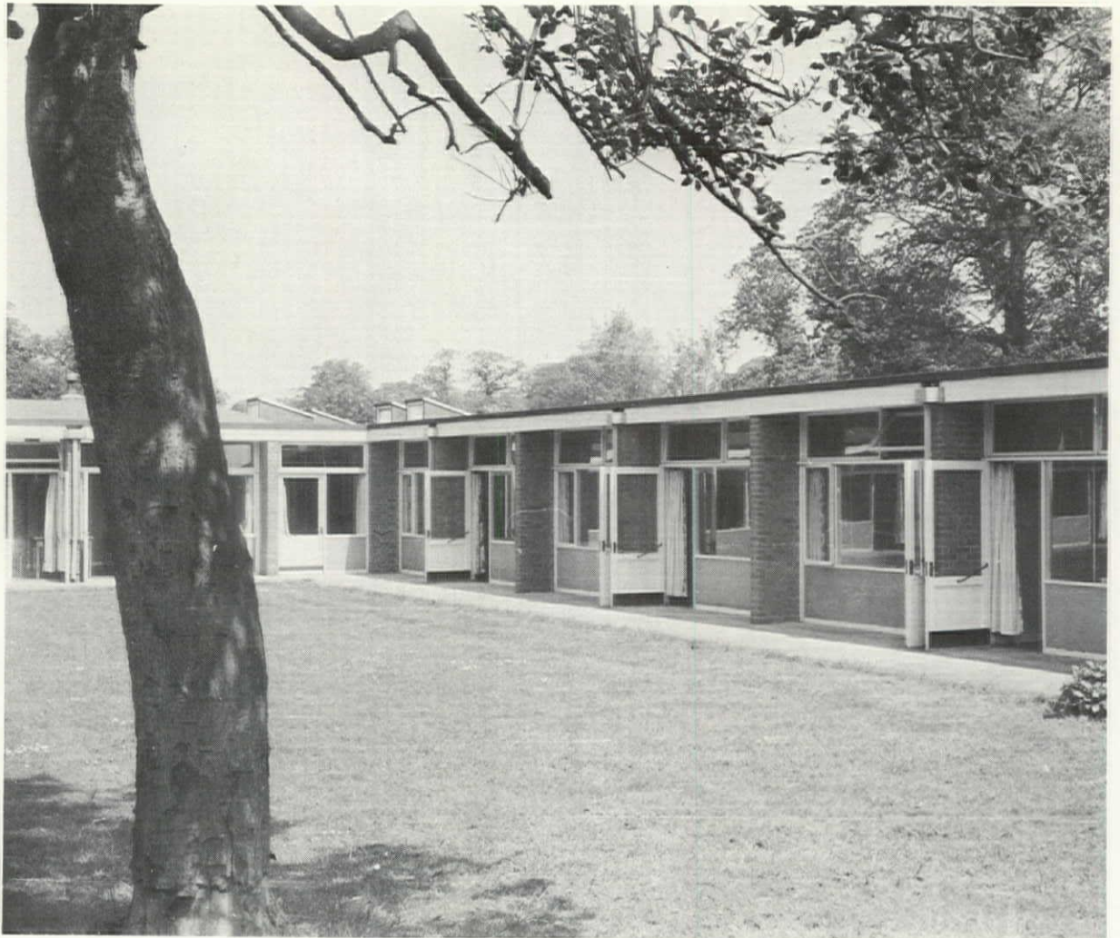
Dormitory, Rehabilitation Center of Queen Elizabeth's Training College for the Disabled, Banstead Place, Surrey, England
