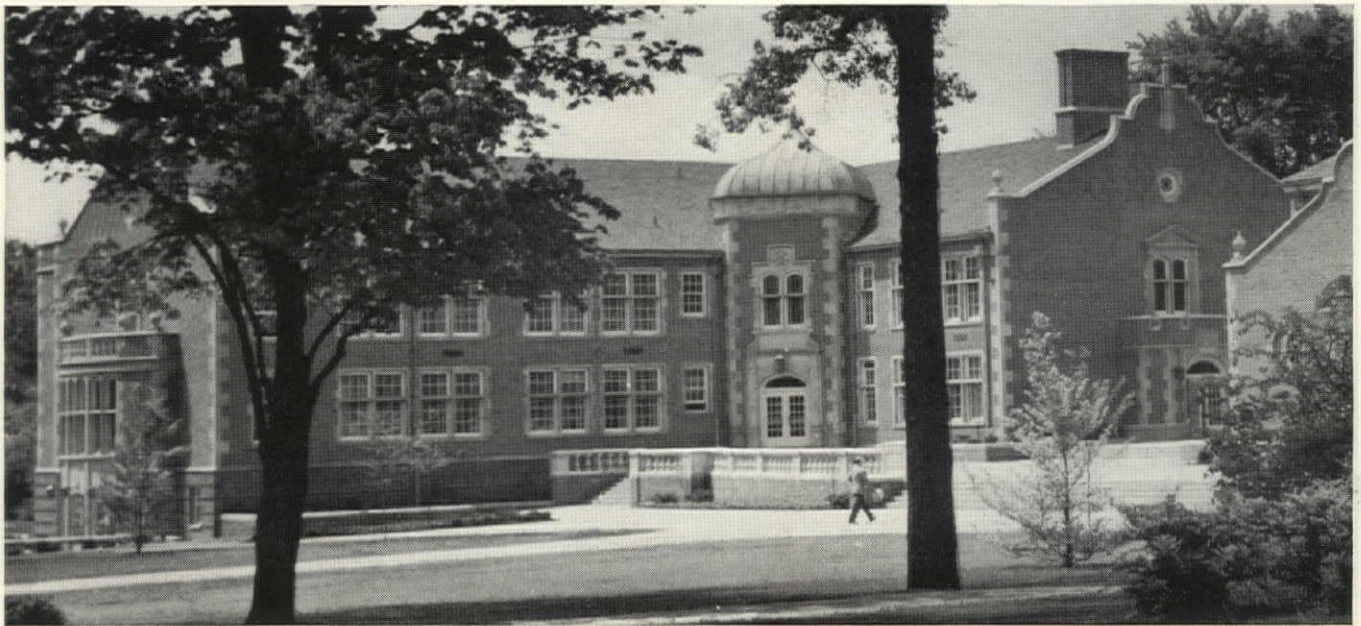
CULVER MILITARY ACADEMY ARCHITECT: WM. B. ITTNER, INC.
