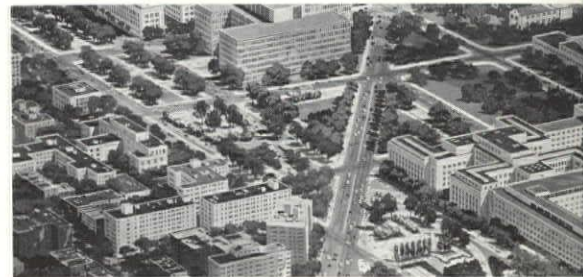
Intersection of Virginia Avenue and proposed "E" Street Expressway cutting through Washington's Federal core. Architects: Satterlee & Smith
