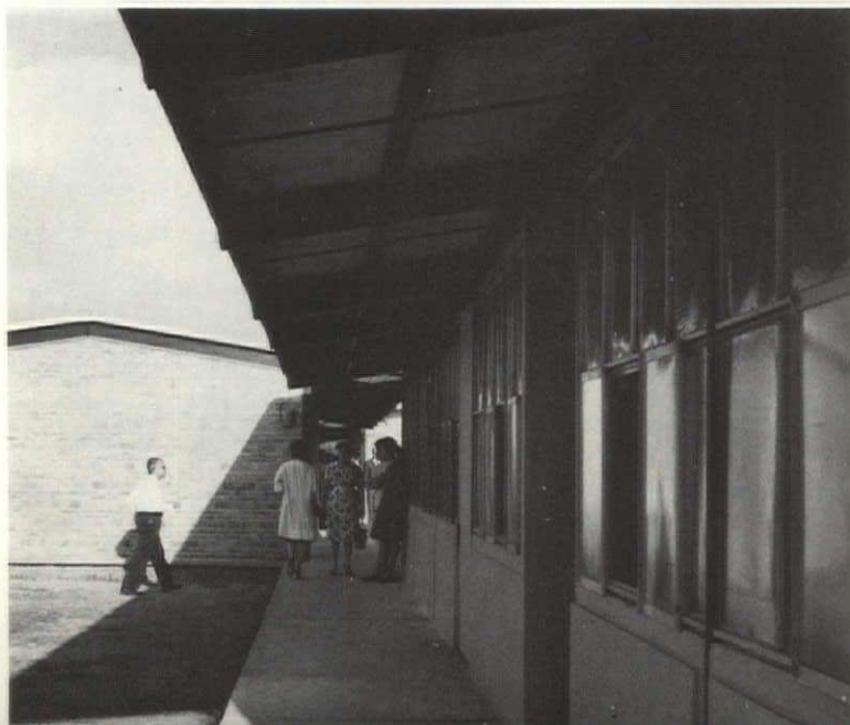
Five-foot overhangs on both sides of building help reduce problem of glare, form protected walkways (see "circulation," p. 103) on floor plan
