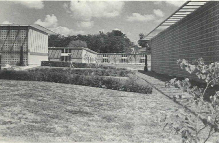
Edward Durell Stone FAIA designed Carlson Terrace buildings to house 200 student families at University of Arkansas, his alma mater. Decorative tile sunscreens form front and back walls. All apartments are two-bedroom, each has private patio or porch
