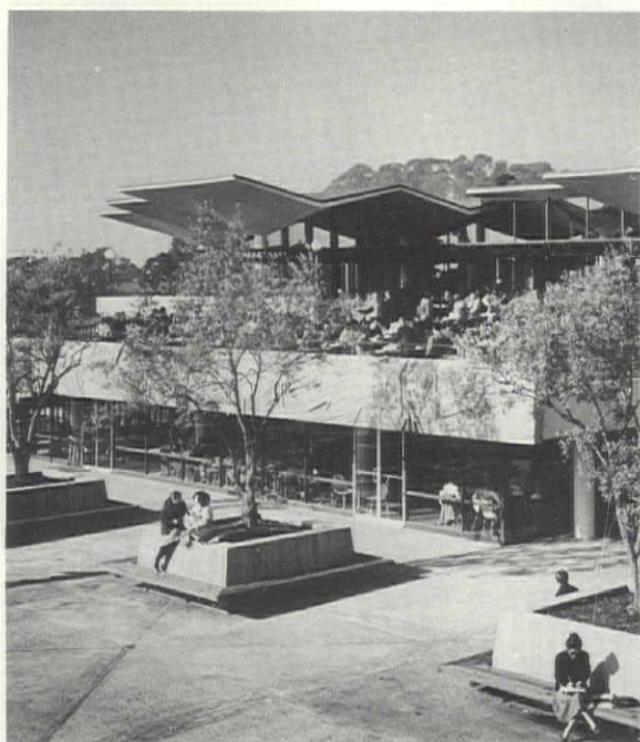
Memorial Hall, college union on Berkeley campus of University of California, has cafeteria facilities for 1000; connects with residence halls by covered passageways. Large portion of cost was financed under College Housing Program. DeMars and Hardison, architects
