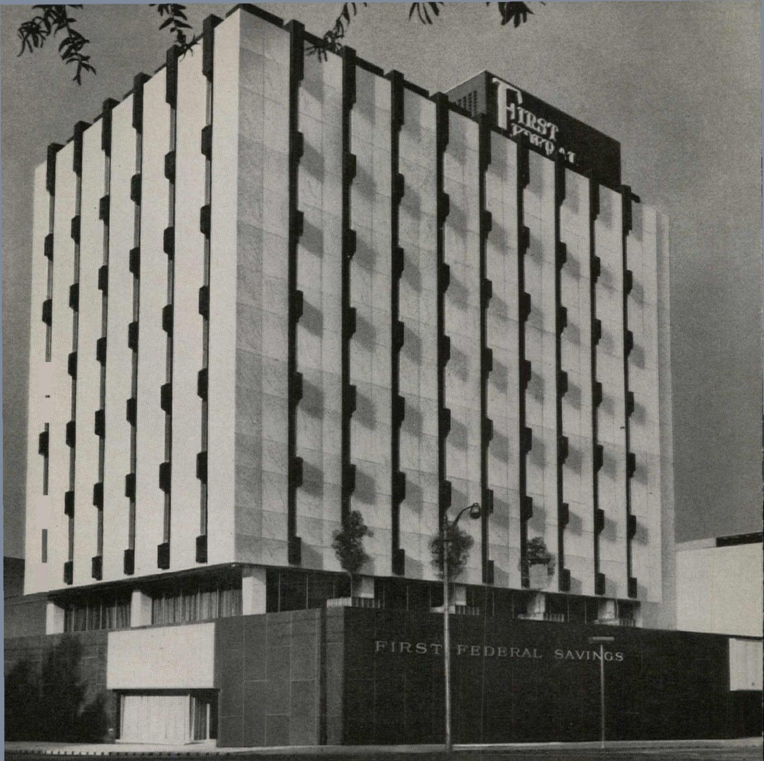
First Federal Savings & Loan Building, Jackson, Mississippi / Architect: R. W. Naef & Associates, Jackson, Mississippi / General Contractor: M. T. Reed Construction Co., Jackson, Mississippi / Material: White Cherokee Georgia Marble, Sand-Rubbed / Winner of Award of Merit—AIA Gulf States Region
