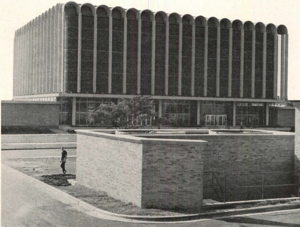
Ceramic Cooling Tower built in August, 1961, at Texas Technological College, Lubbock, Texas. Two Cells: 3,520 GPM; Specifications °F: 100-85-74. Architects: Davis, Foster, Thorpe and Associates, Inc., Architects and Engineers, El Paso, Texas; Consulting Engineers: Zumwalt & Vinther, Engineers, Dallas, Texas.
