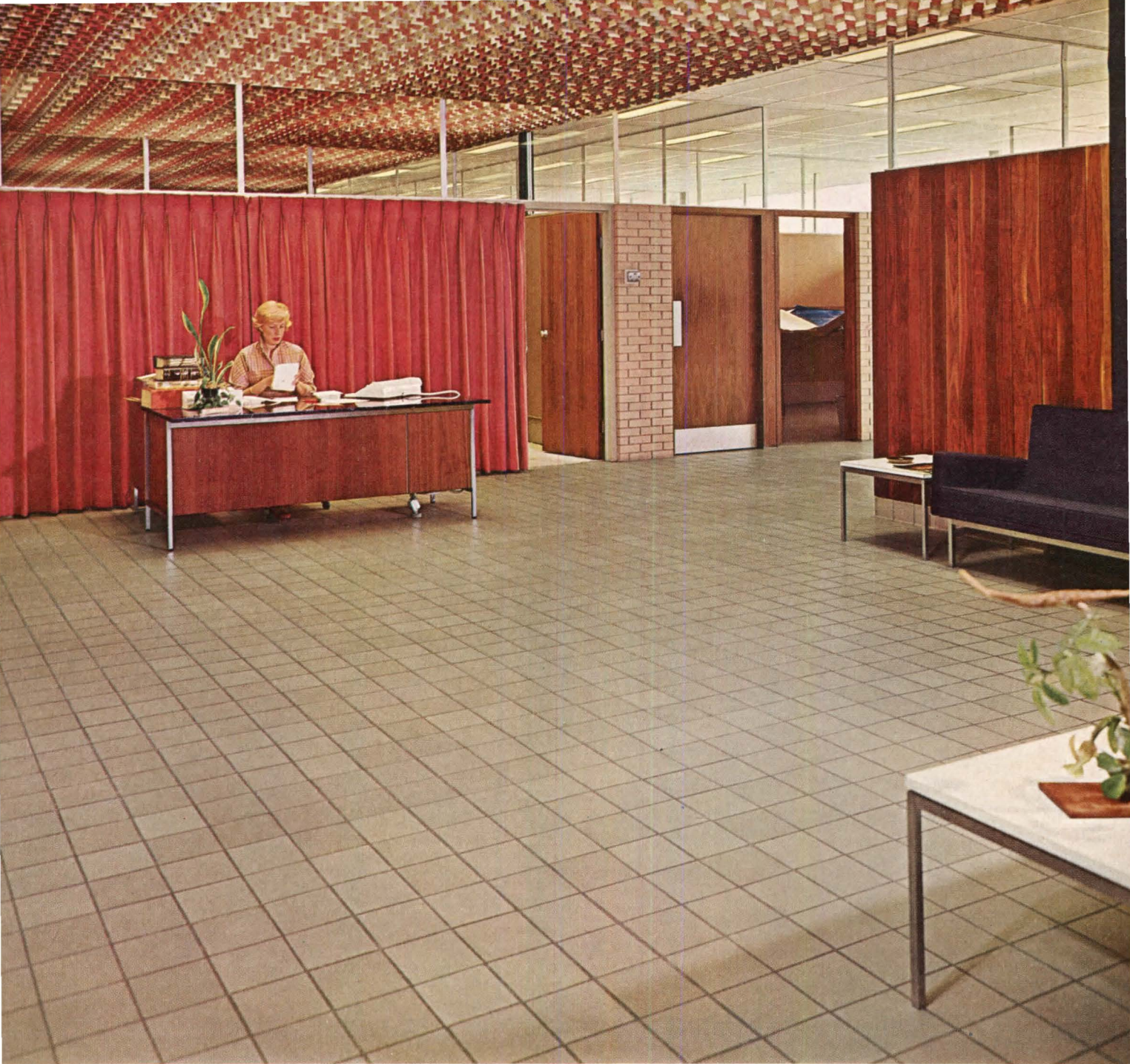
Robert E. Lamb, Inc., Valley Forge, Pa. Murray quarry floor is 6" x 6" x 1/2", Fawn Gray. Architect: Jules Gregory. Tile Contractor: Wissahickon Tile Company. Plate 510.
