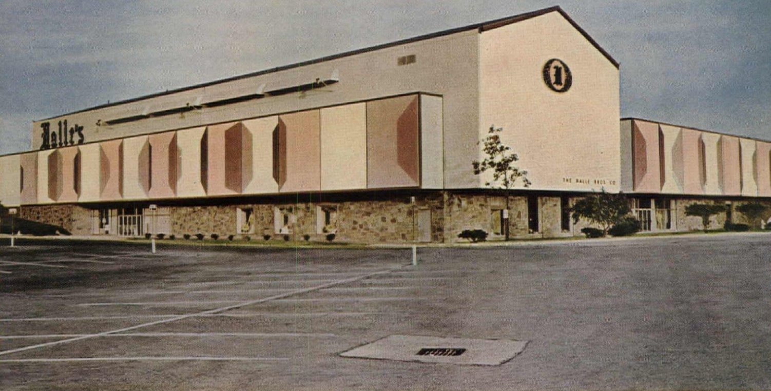
The Halle Bros. Co. Westgate Suburban Store Greater Cleveland. Design Coordinator: Pierre Lalire. Planners and Designers: Raymond Loewy / William Snaith, Inc.; Architects: Fordyce & Hamby. Says John G. Mitchell, Operating superintendent of the Halle Bros. Co.: "We didn't repaint until 10 years after the first coat of Colorcoat went on."
