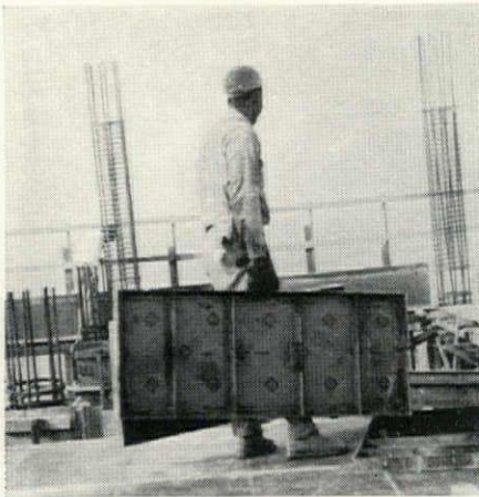
SYMONS SLAB SHORE CUTS DECK TIME FROM 5 TO 4 DAYS
