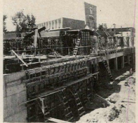
UNIQUE SLAB FORMING PLYWOOD PANS AND PRE-FAB SHORING SYSTEM
