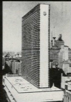
NEW YORK HILTON William B. Tabler, Architect
