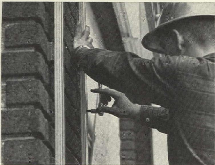
Vertical struts are anchored to existing facade.
