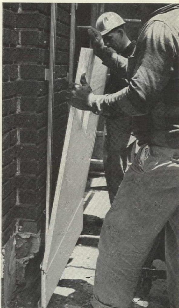
Horizontal members lock into grooves in edge of marble.
