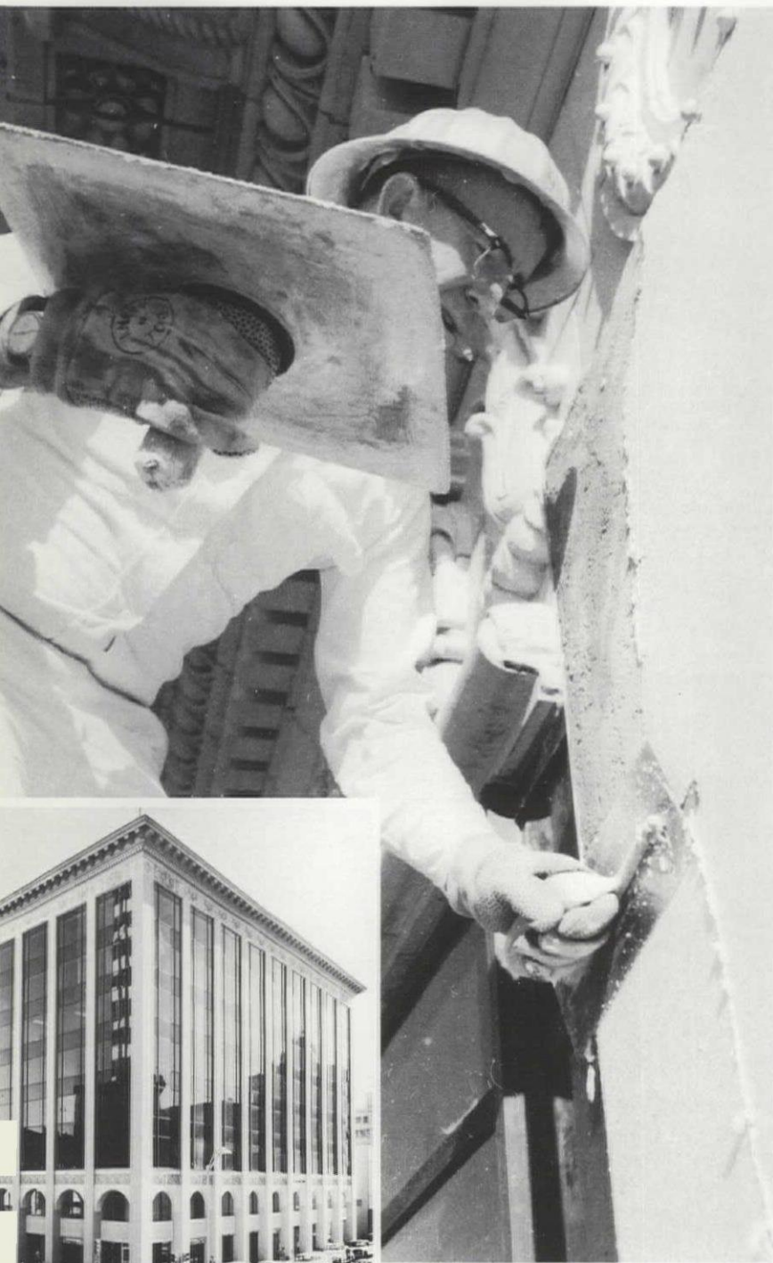
El Paso International Building Garland & Hillis, Architects LARSEN GRANITE FINISH Applicator: Carter Lathing & Plastering Co.
