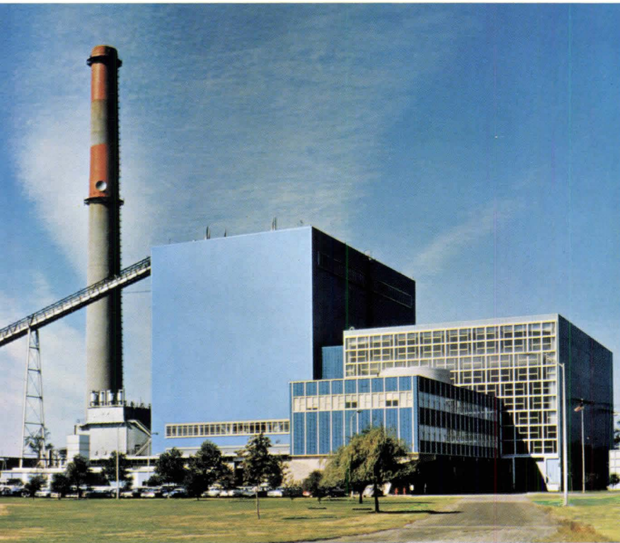
CONNECTICUT LIGHT & POWER CO., South Norwalk Harbor, Conn.; Kahn & Jacobs, Consulting Architects; United Engineers and Constructors, Inc., Engr. and Contractor.
