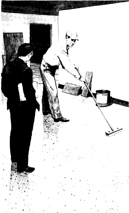
Seals new terrazzo for protection during construction
