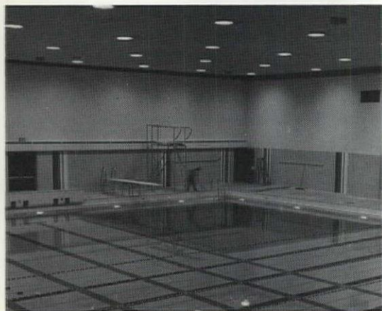
Natatorium is 106' x 141'. Moisture condensation is no problem because of Behlen's all-steel Roof-Ceiling System. The steel ceiling is a highly efficient vapor barrier. Insulating materials are poured above the ceiling chord to provide superior thermal value.
