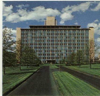
Advanced look of UFG Headquarters, Charleston, W. Va., is complemented beautifully by modern Kentile Floors.
