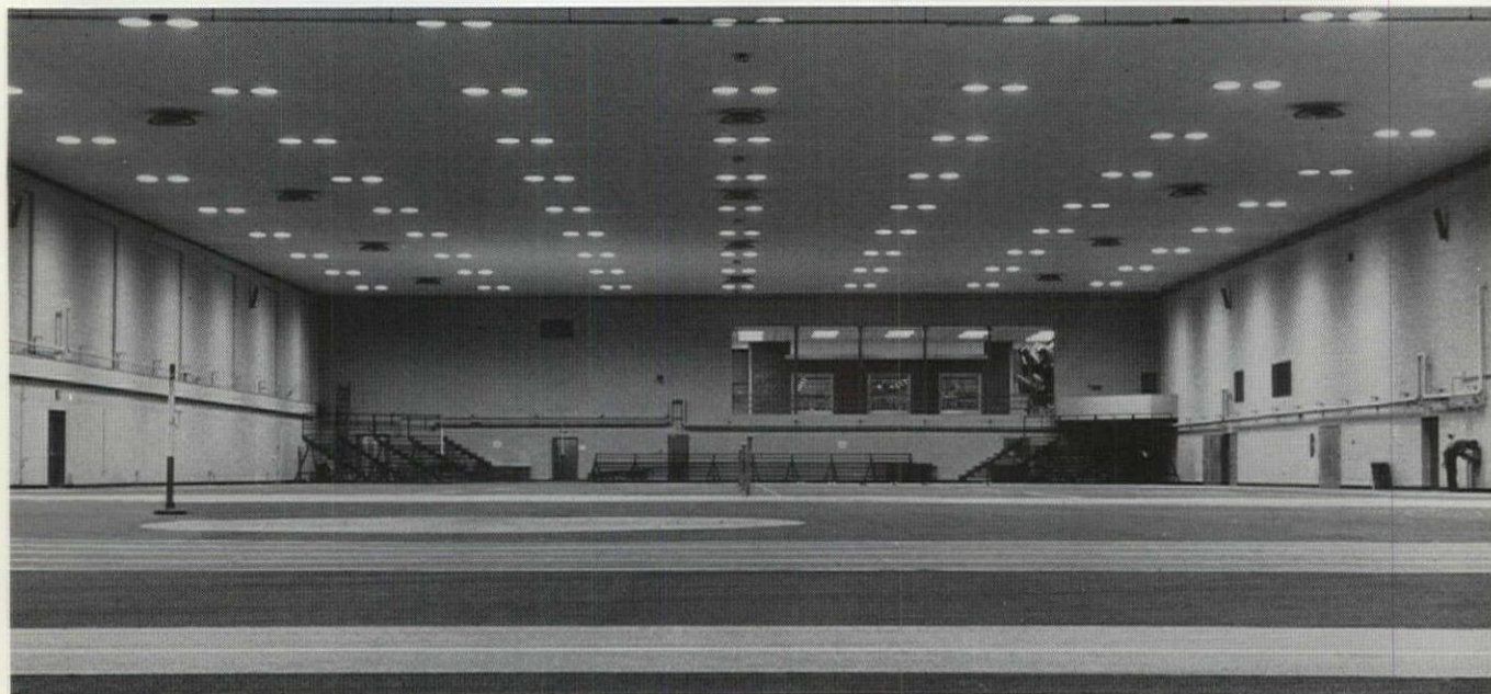
Architect: Richard Hawley, Cutting and Associates, Cleveland, Ohio. Ceiling and roof are combined in same system in 131' x 349' gymnasium.
