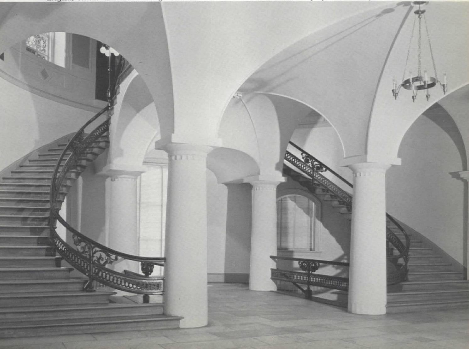
Elegant, cantilevered staircases greet the visitor inside south entrance, sweep up to the third-floor Marble Hall.
