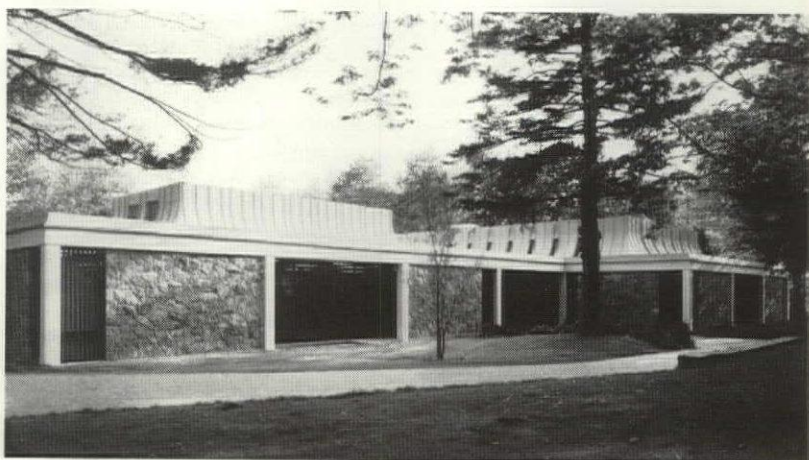
Mt. Pleasant Public Library, Pleasantville, N. Y. Arch: Gibbons and Heidmann, White Plains, N. Y.
