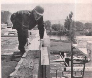
Pre-formed flashings were easily positioned prior to joining.
