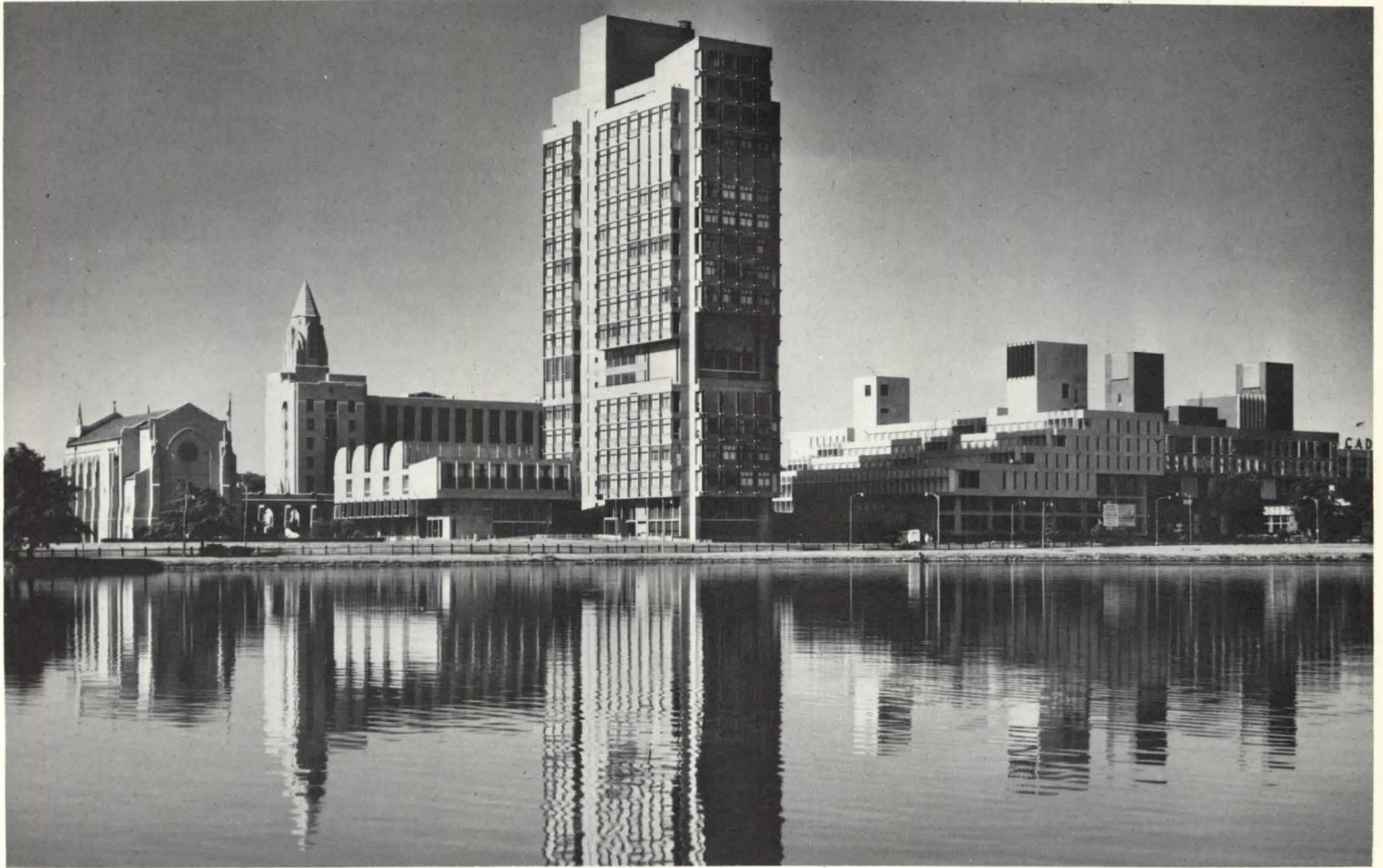
Boston University Campus, whose new buildings share an interlocking vocabulary while still acknowledging the patina of some older ones.
