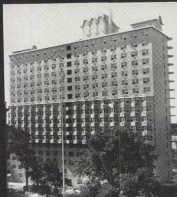
ISABELLA HOUSE (Elderly Housing) N. Y. Joseph Douglas Weiss, Architect
