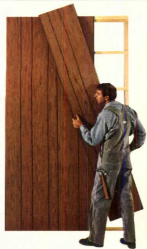
The One-Man Paneling. One man can panel a room by himself with 16"-wide Marlite Planks.
