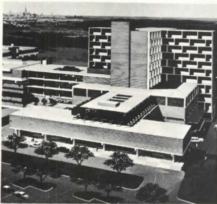
Bexar County Teaching Hospital, San Antonio, Texas. Equipped with Security doors and automatic cart handling system. Dumbwaiters by Otis.
