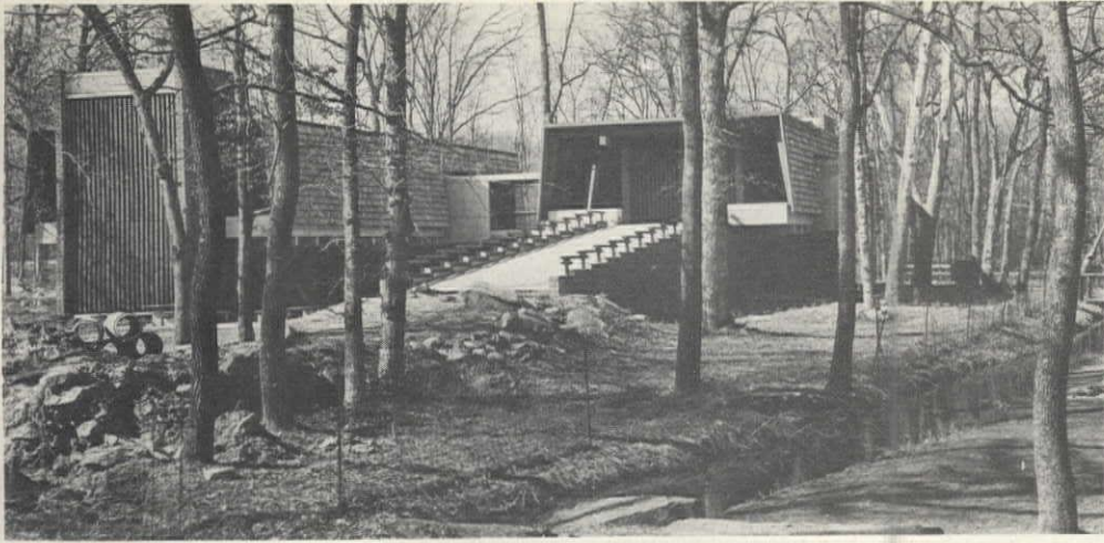
In the Visitor Center ('68) in Great Falls Park in Virginia, W. Kent Cooper, AIA, has linked the two buildings — one for exhibits, the other for movies — by a covered passageway.
