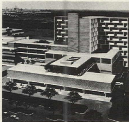
Bexar County Teaching Hospital, San Antonio, Texas. Equipped with Security doors and automatic cart handling system. Dumbwaiters by Otis.
