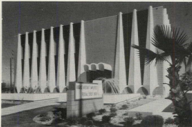
Hughes Aircraft Employees Federal Credit Union. Perry C. Langston, Architect.
