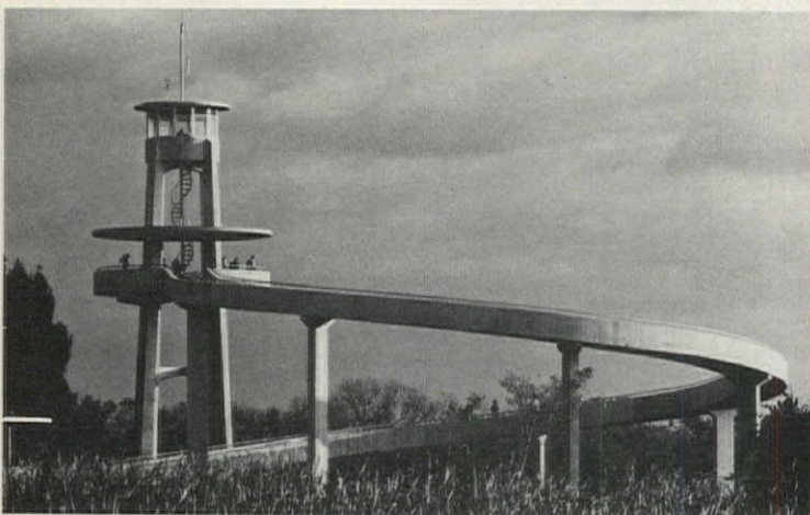
The Everglades National Park in Florida includes the Parachute Key Visitor Center ('61) and the Shark Valley Observation and Fire Tower ('65), both developed by the National Park Service staff.
