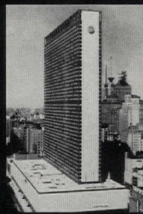
NEW YORK HILTON William B. Tabler, Architect
