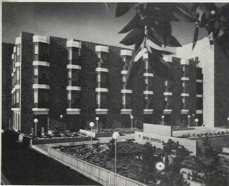
The environmental needs of the community come into proper perspective when the architect is involved in community questions. Encino Hospital (Howard R. Lane Associates) accommodates the public with a plaza.
