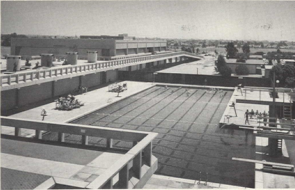
Cypress College Phase I , Cypress, California. New Facilities. Architects: Caudill Rowlett Scott; William Blurock & Partners.
