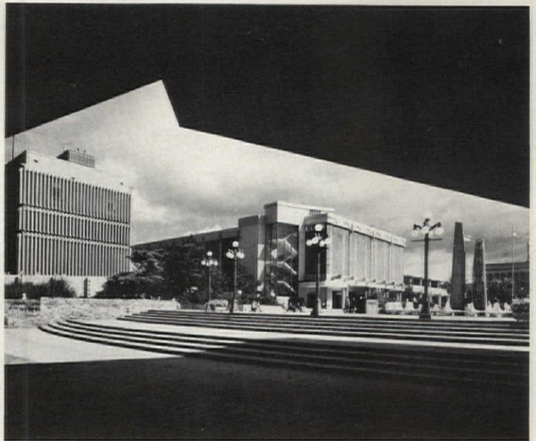
The visitor who enters the square from the Government Street entrance is aware of a true "explosion of space" effect, almost baroque in manner. The severely articulated elevation of the police department building is an excellent foil for the thick and colorful planting below.
