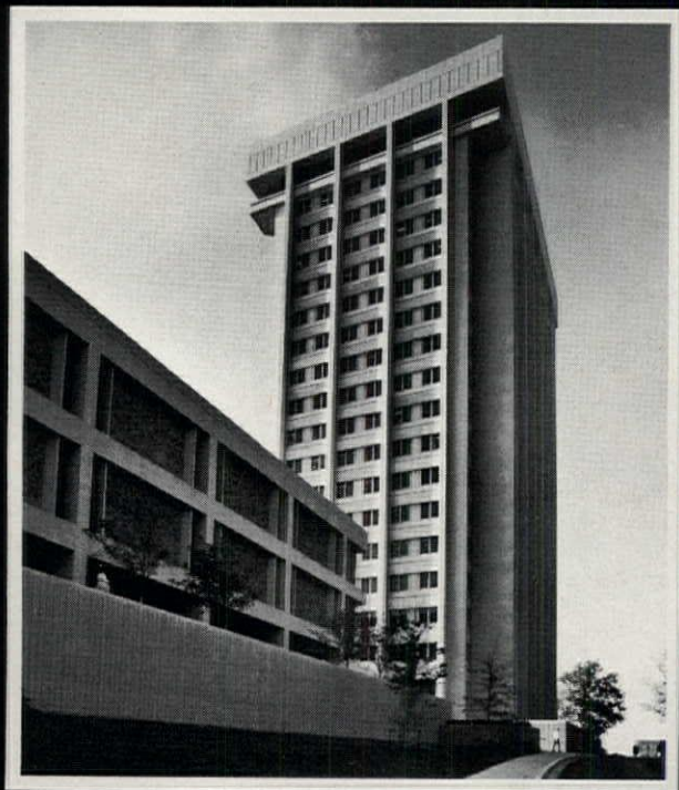
(Above) Patterson Office Tower and White Classroom Building. Architects: Johnson-Romanowitz, Lexington. General Contractor: Foster & Creighton Company, Lexington. Six Dover gearless traction elevators with Computamatic IV Control.
