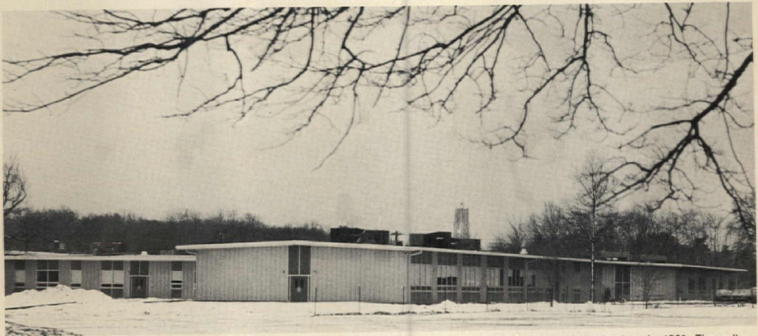
Temporary facilities at Bergen Community College, Paramus, New Jersey, started with one 25,000 square foot structure in 1968. The college placed a 28,700 square foot addition in 1969. The building layout was prepared by the owner/architect, The Grad Partnership (then Frank Grad & Sons); bids were advertised and lowest bidder selected. The successful bidder engineered the structural, mechanical and electrical (with the architect's approval). The lump sum bid was a complete turnkey job, including financing. The college had a year-by-year option of purchasing the buildings and in both cases did so the first year. Had they not been sold after 10 years, they would have been removed and the site restored.
