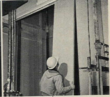
2. Installing core panel.
