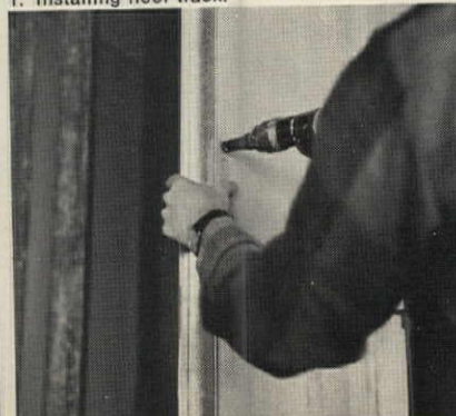
3. Attaching core to T-spline.
