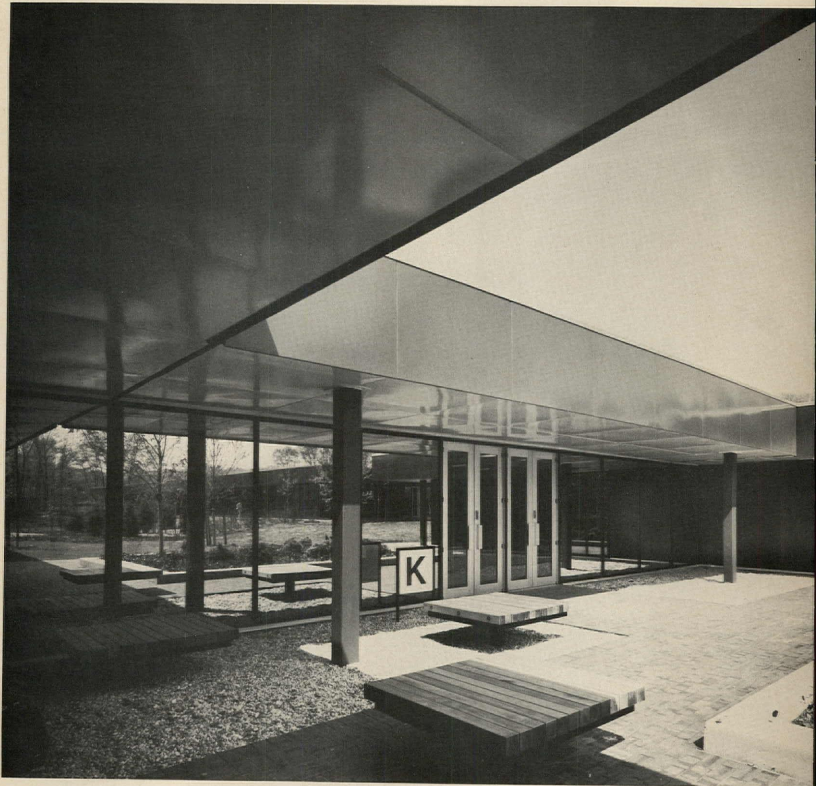
The South Campus Surge Buildings, State University of New York at Stony Brook by Smith, Hinchman & Grylls Associates, Inc. prove that permanent quality facilities for temporary use need not convey an air of temporariness. The State University Construction Fund developed the complex.
