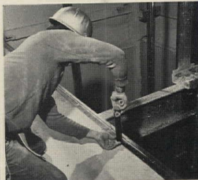
1. Installing floor track.
