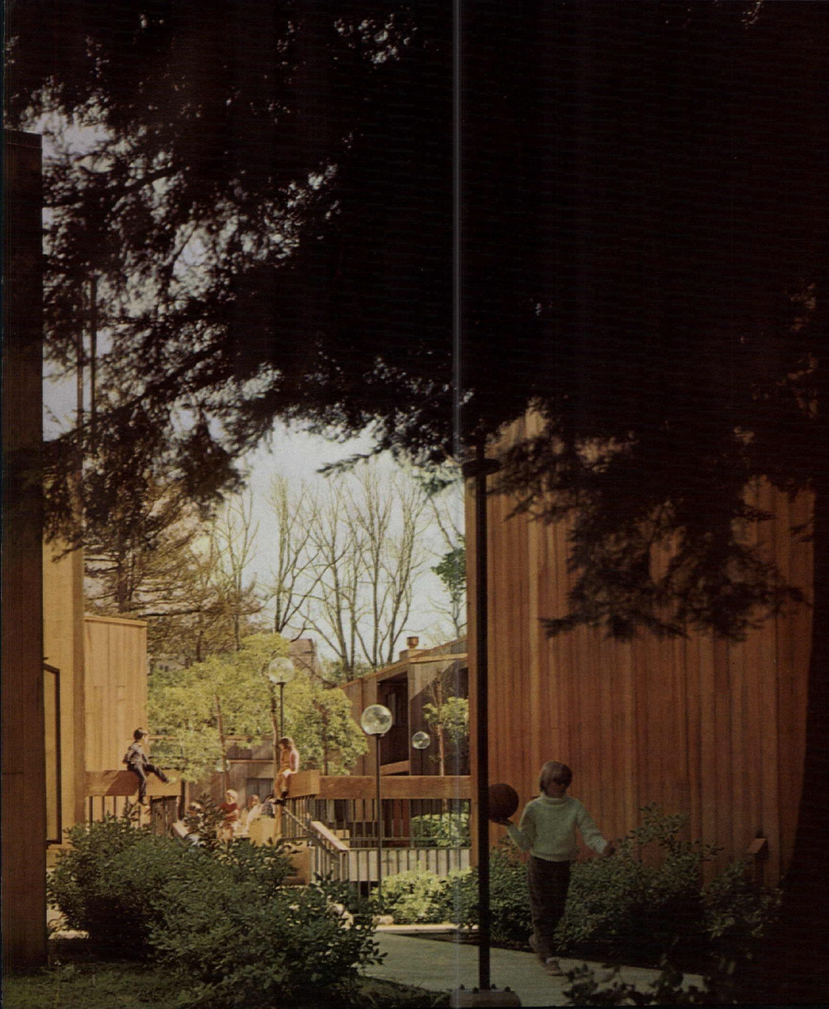
Married student housing, Theological Seminary, San Anselmo, California Architects: Frants Albert, AIA and Wm. M. Abend, AIA, San Francisco
