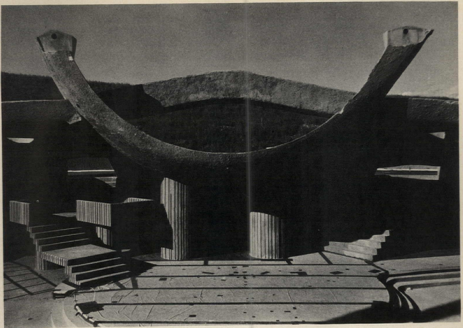
Soleri-designed Outdoor American Indian Theater in Santa Fe, with Pacheco & Graham as project architects, seats 2,000 spectators. The concrete forms were cast on earth with earthmoving equipment and hand finished. After the concrete had cured, the earth was removed from beneath.
