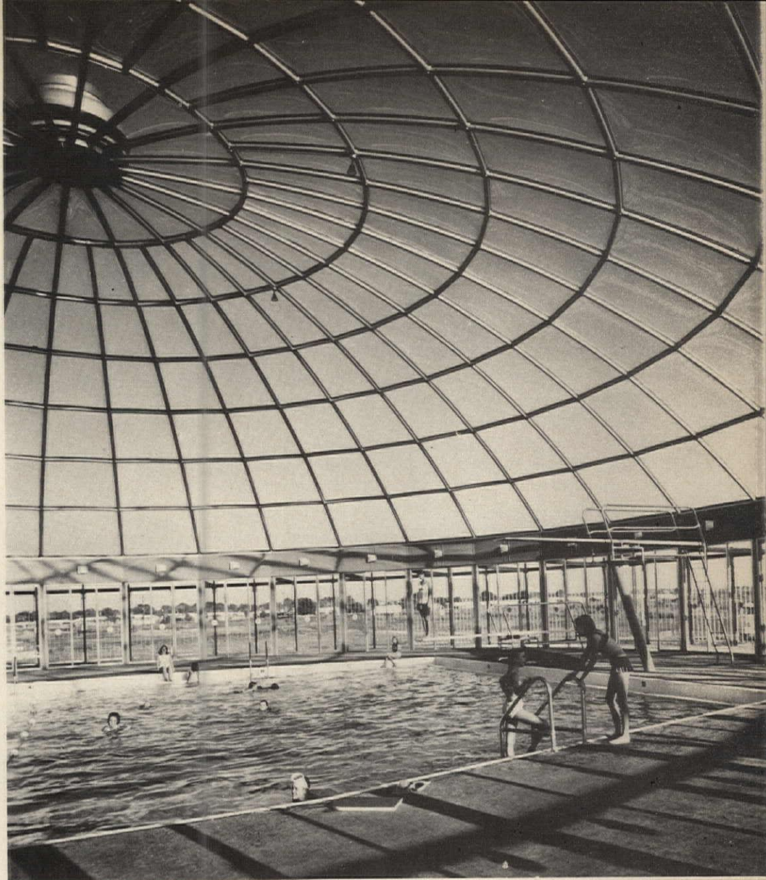
Designed by Aycock & Neville and appropriately named the Aquadome, this pool in Decatur, Alabama, gives children a year-round facility. The dome is of acrylic plastic.
