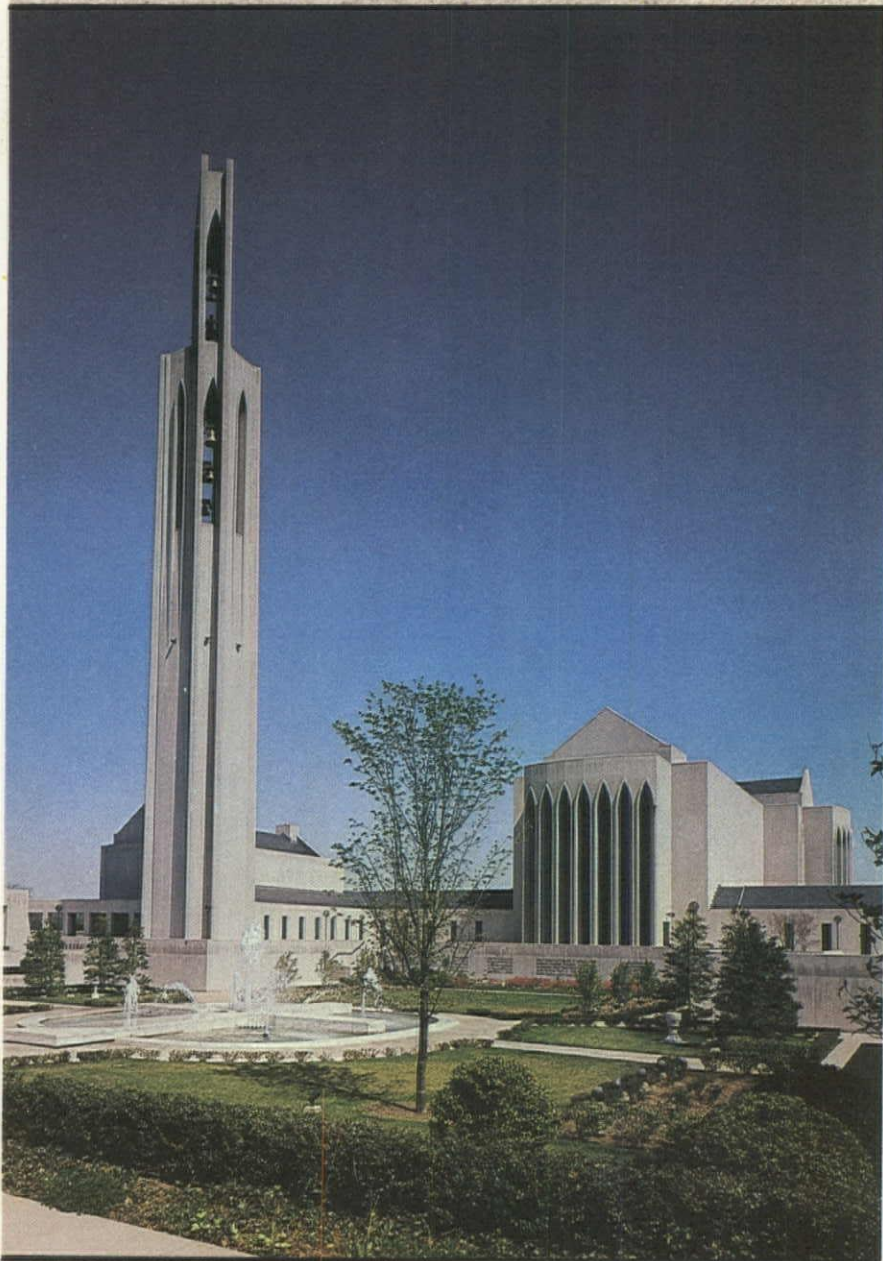
THE NATIONAL PRESBYTERIAN CHURCH AND CENTER, Washington, D. C. winner of the Building Stone Institute Award of Merit, Harold E. Wagoner & Associates, architects.
