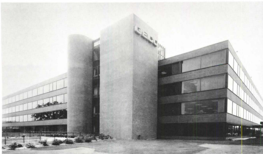
Three existing outboard "cores" will be joined by two more when new wing is added.
