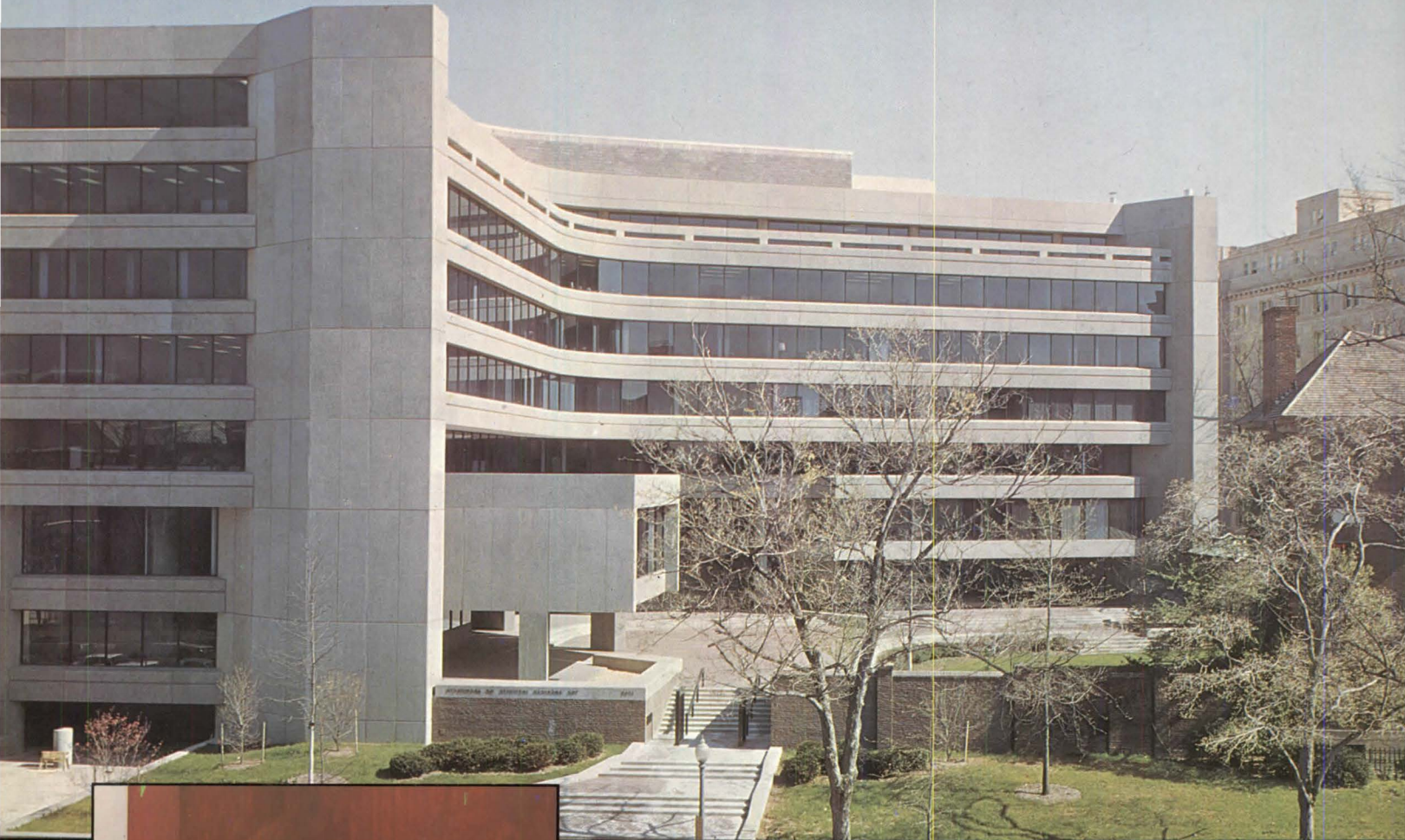
A.I.A. HEADQUARTERS BUILDING, Washington, D.C. — The Architects Collaborative
