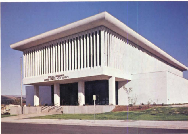
Georgia Brilliant was selected for the new Post Office and Federal Office Building in Wenatchee, Wash. Architects: Warren Cummings Heylman & Associates, Spokane, and Fraley & Leighton, Wenatchee. Erector: Blaesing Marble Co., Beaverton, Ore.
