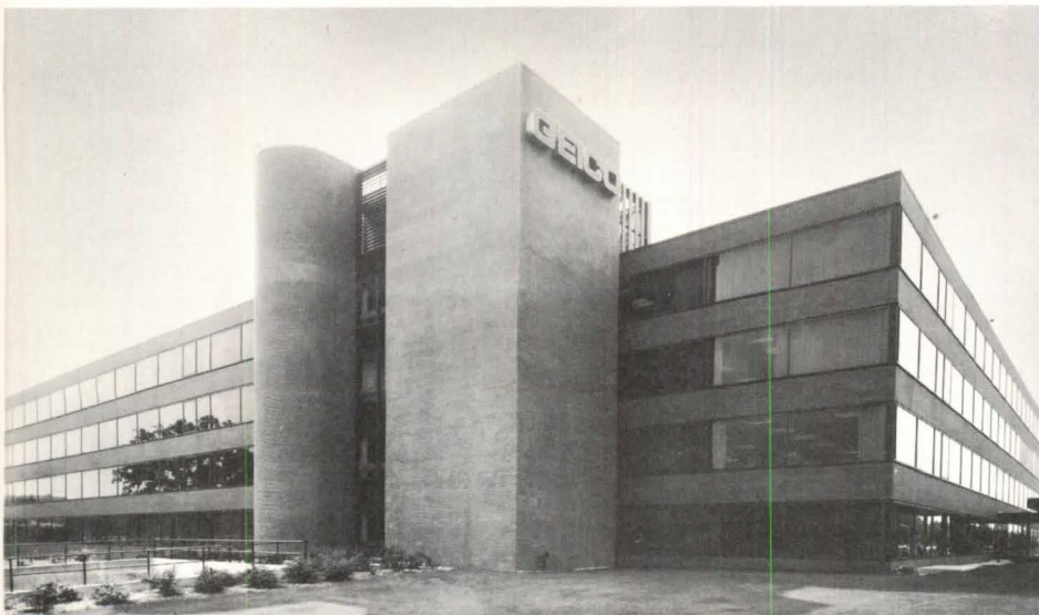
Three existing outboard "cores" will be joined by two more when new wing is added.
