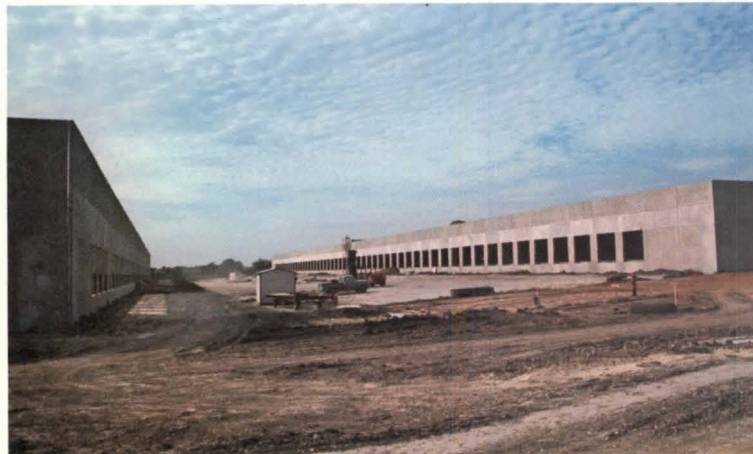
Ease and speed of erection with Vulcraft products enabled the first building to be under roof in 19 days.
