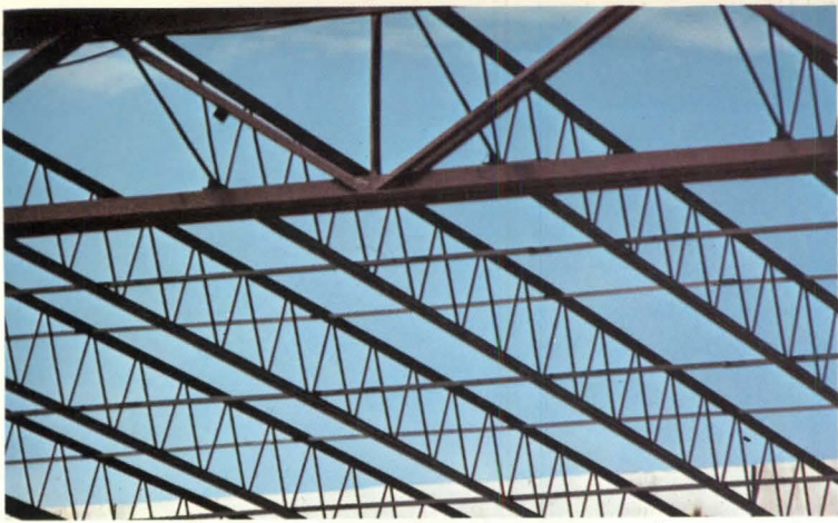
Open web design allows ducts, pipes and wiring to pass directly through the steel members.
