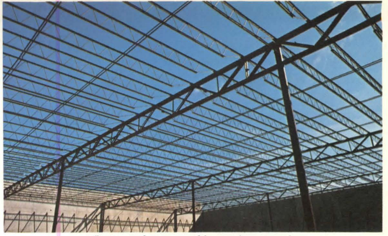
Increased spans and larger bays result from computer design of joists and joist girders.
