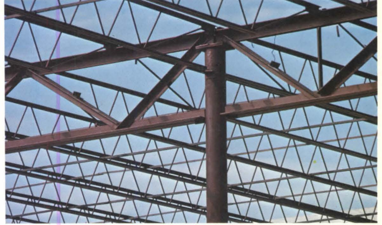
Lighter weight columns can oftentimes be used with joist girders. And that's a big advantage.
