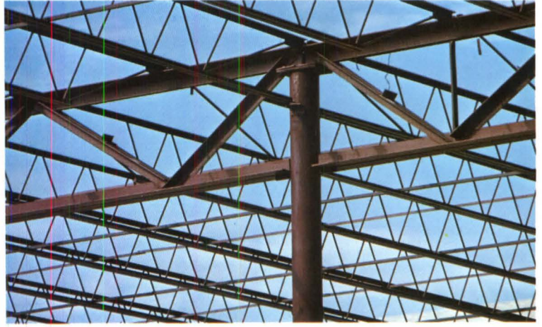
Lighter weight columns can oftentimes be used with joist girders. And that's a big advantage.
