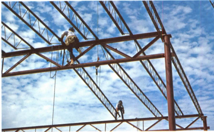
The simplicity and light weight of Vulcraft joists and joist girders make erection fast and easy.
