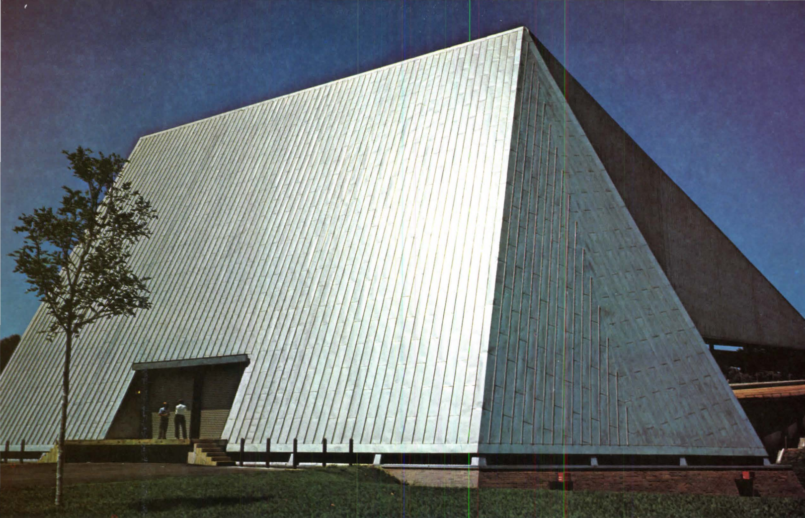
Robin Hood Dell West, Philadelphia, Pa. • Architects: John H. MacFadyen and Alfredo De Vido, New York • Associate Architect: I. Demchick, Philadelphia, Pa. • Roofing Contractor: Warren-Ehret-Linck, Philadelphia, Pa.
