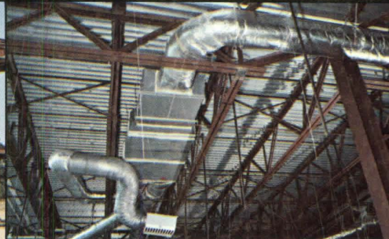
Vulcraft joists and joist girders can be designed to easily accommodate all lighting, heating, air conditioning, wiring, duct and pipe requirements.
