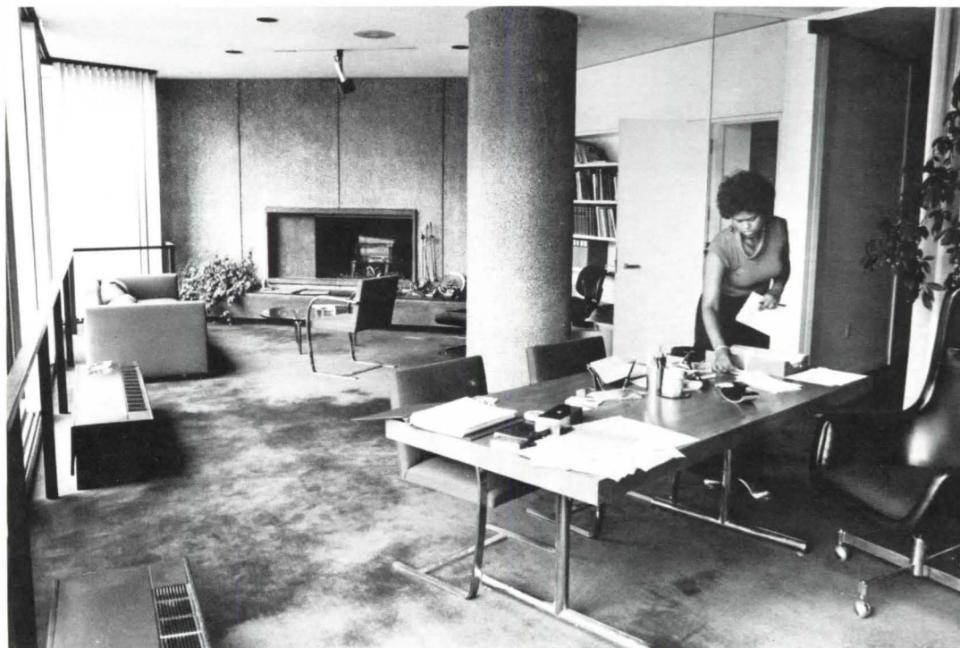
The second floor landscape (top) now ends at two glazed, offices. Above, the executive vice president's office.
