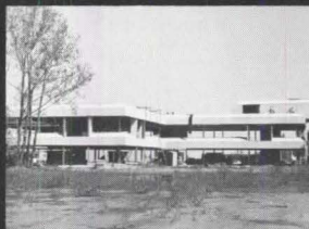
Aggregate faced panels in a variety of sizes from 3' x 3' to 12' x 9' for a MetroCenter office building, Nashville, Tenn. Architect: Hart, Krivatsy & Stube, New York, N.Y. Manufacturer: Cem-Fil Corporation, Nashville, Tennessee.
