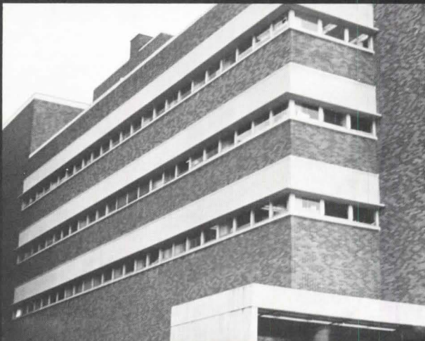
Sun Shades, University of Washington. Architect: Shavey & Schmidt. Manufacturer: Olympian Stone Co., Redmond, Washington.
