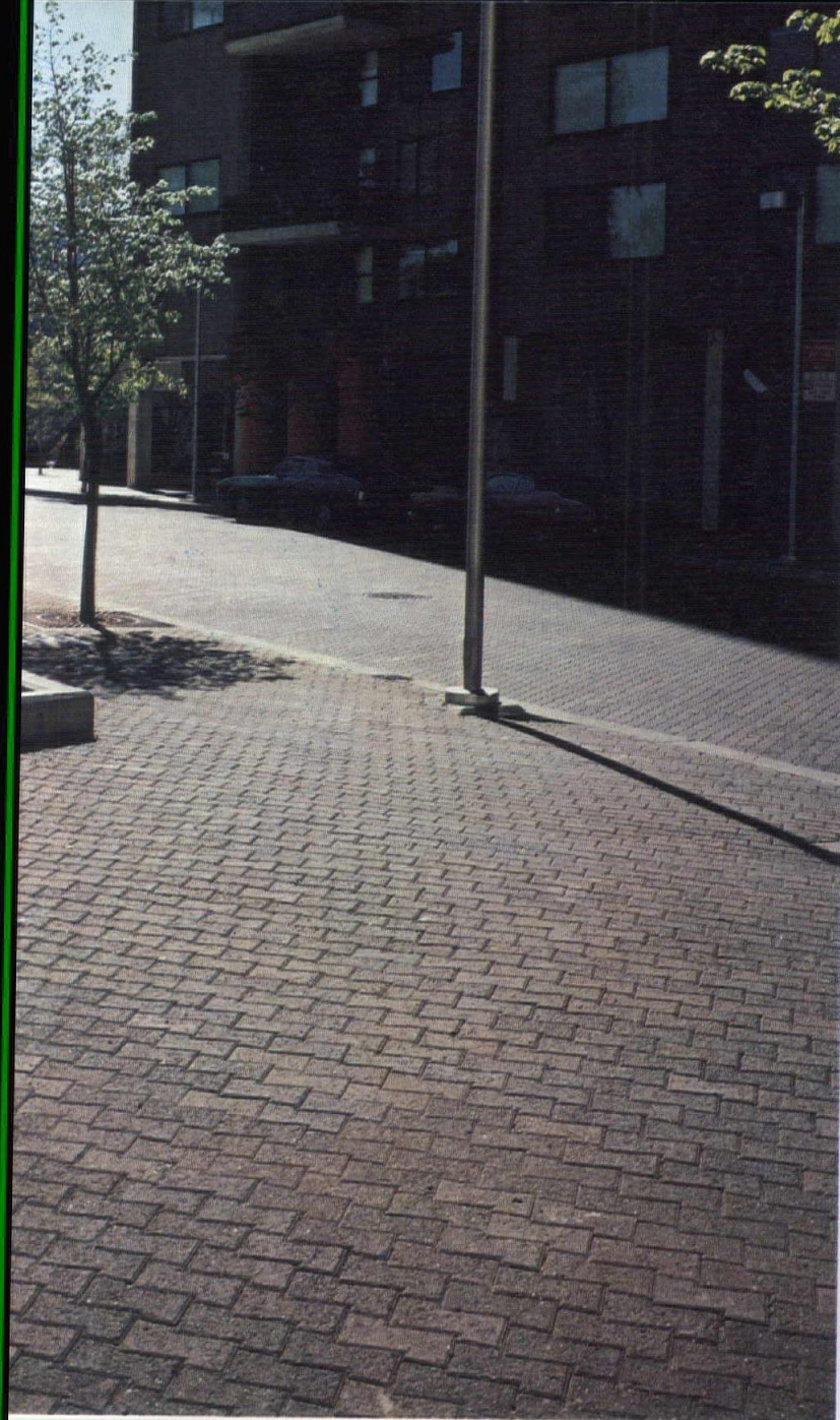
Roosevelt Island, New York City. This new town in the East River uses Concrete Pavers over a total area of 4½ acres for both pedestrian and vehicular traffic. Installation has been in use since 1972. Zion & Breen Associates, Landscape Architect & Site Planners.
