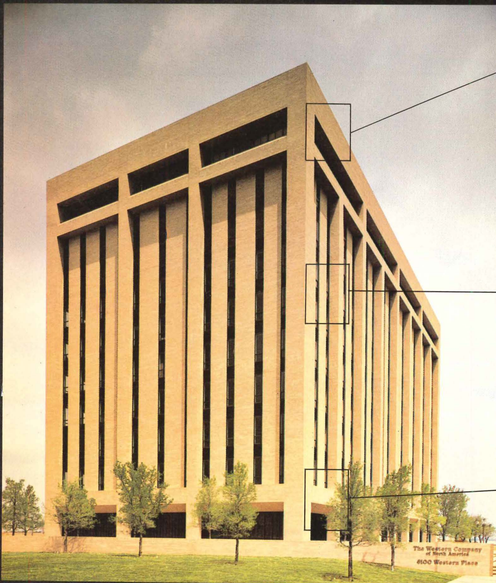
Hung soffit panels constructed of Acme Brick and bond mortar produce deep, shadowed recesses beneath the parapet.
