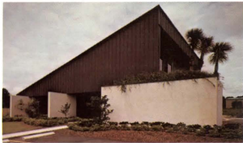
Architect's Office Gainesville, Florida Architect: John Don Puckett Gainesville, Florida
