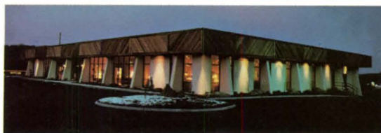
Fowler Brothers Furniture Store Knoxville, Tennessee Architect: James R. Johnson & Associates Knoxville, Tennessee
