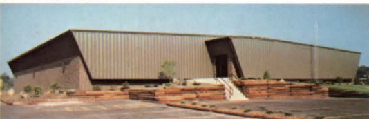
Century Harbor Racquetball Club Middleton, Wisconsin Architect: Douthitt Associates, Inc. Madison, Wisconsin
