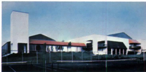
Columbus Indoor Tennis Club, North-Oak Creek Gymnastics Academy-Columbus, Ohio Architect: Acock White and Associates-Columbus, Ohio
