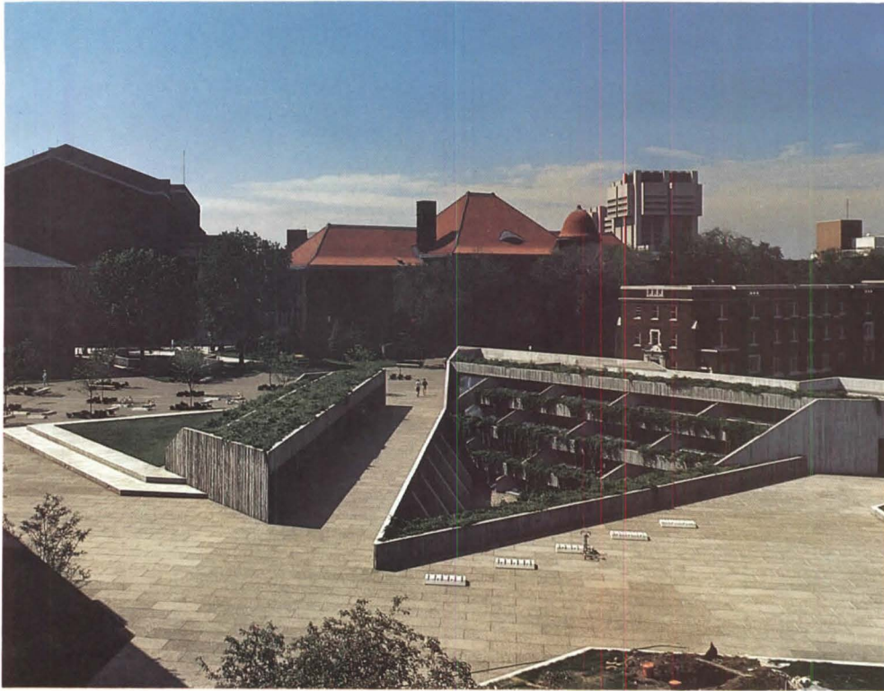
Previous page, top, the south facade of the Western Life Insurance Co., Woodbury, Minn., by Ellerbe, Inc., steps forward to let each floor shade the one below. Previous page, below, Steve Baer's own house near Albuquerque is a 'zome' (asymmetrical faceted dome) with windmill. Left, the University of Minnesota's Williamson Hall bookstore by Myers & Bennett is almost completely underground, preserving important campus open space. Right, Fuller Moore's own house with solar collector, near Oxford, Ohio. Right below, in the Maine countryside, Roc Caivano's passively heated house with Trombe wall.
