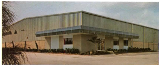
Georgia Pacific Corp. Distribution Div. Baton Rouge, Louisiana Architect: Pesce Clendening Associates Dallas, Texas
