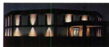
Westland Medical Center Wichita, Kansas Architect: Howard V. Harrison Wichita, Kansas
