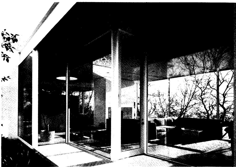
House on the lake, Glencoe, Ill.; Booth Nagle & Hartray/Ltd., Chicago (above). The house, situated on a bluff overlooking Lake Michigan to the northeast and a ravine to the northwest, is built into a hill, which helps compensate for heat loss through large glass areas. The children's bedrooms and a large playroom are on the lower level; the upper level is a one-bedroom adult living loft space. The jury commented, "It's so technically advanced—and it's such an anachronism in terms of today's architecture. We have to see it as a terrific curatorial effort. It's so sincere; so perfectly done." Philip Turner, photographer.
