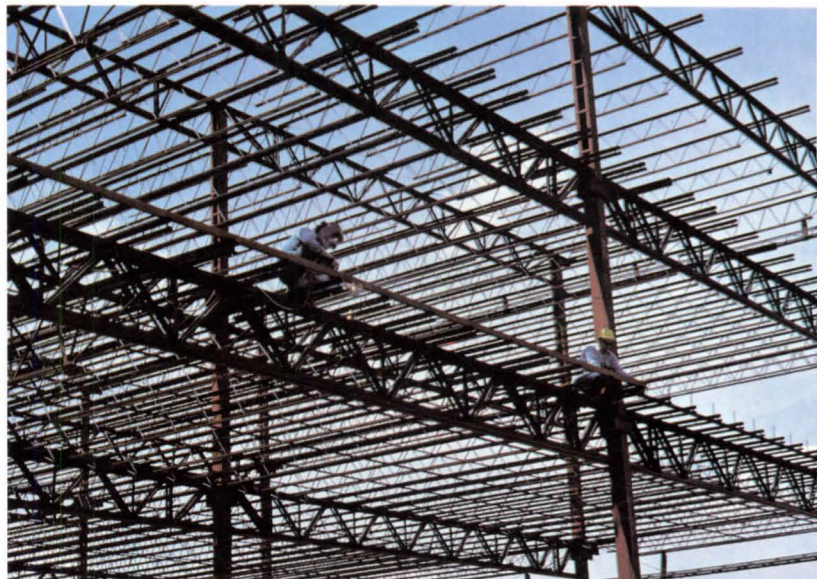
The simplicity and light weight of Vulcraft joists and joist girders make erection fast and easy.
