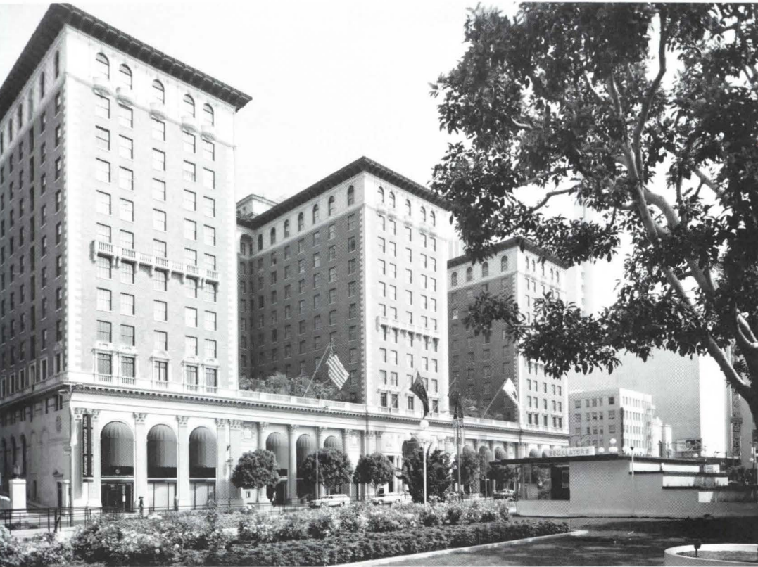
Restoration of the exterior (left) included tuck pointing, acid washing of masonry, epoxy injection on terra cotta and repair of wooden double-hung sash. On the interior (below) cast plaster was used for the repair of ornamentation.
