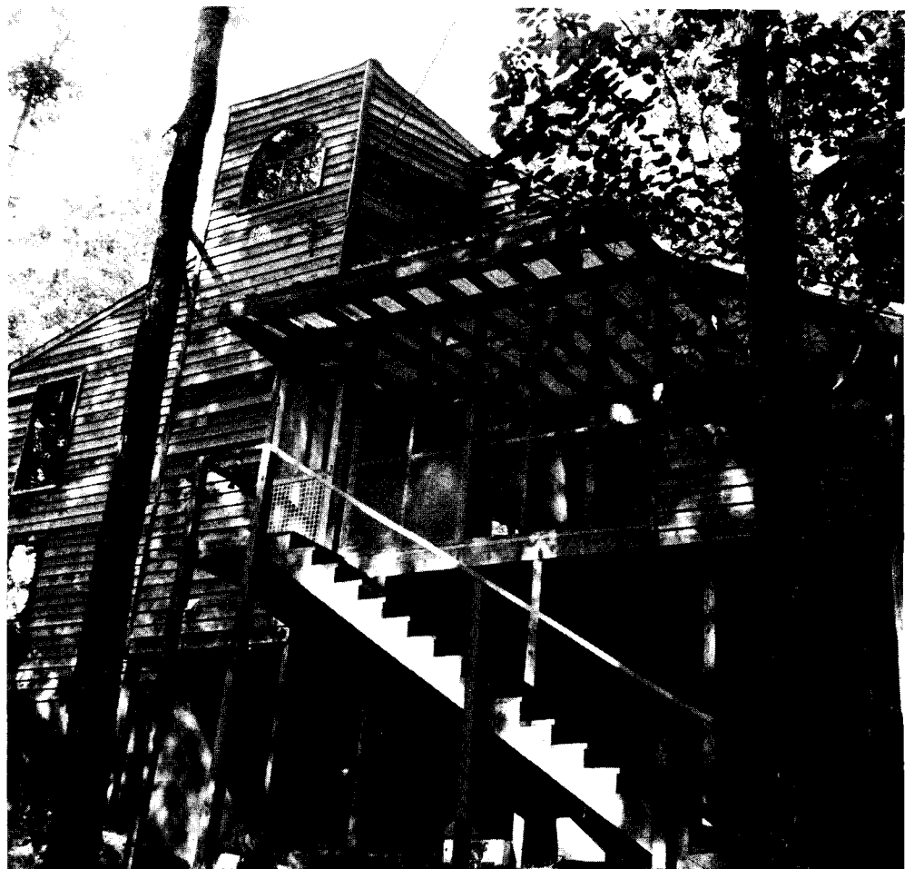
Louisiana Architects Association. David Burrus Boathouse, New Orleans; Lyons & Hudson, New Orleans (left). The architect incorporated the existing frame building into the new design. The two-story glass-enclosed entry area is the main focal point. The roof framing was changed, lending spatial variety and emphasis to the component parts of the building. Major living spaces were rearranged to capitalize on the views to the marina. Frank Lotz Miller, photographer.
