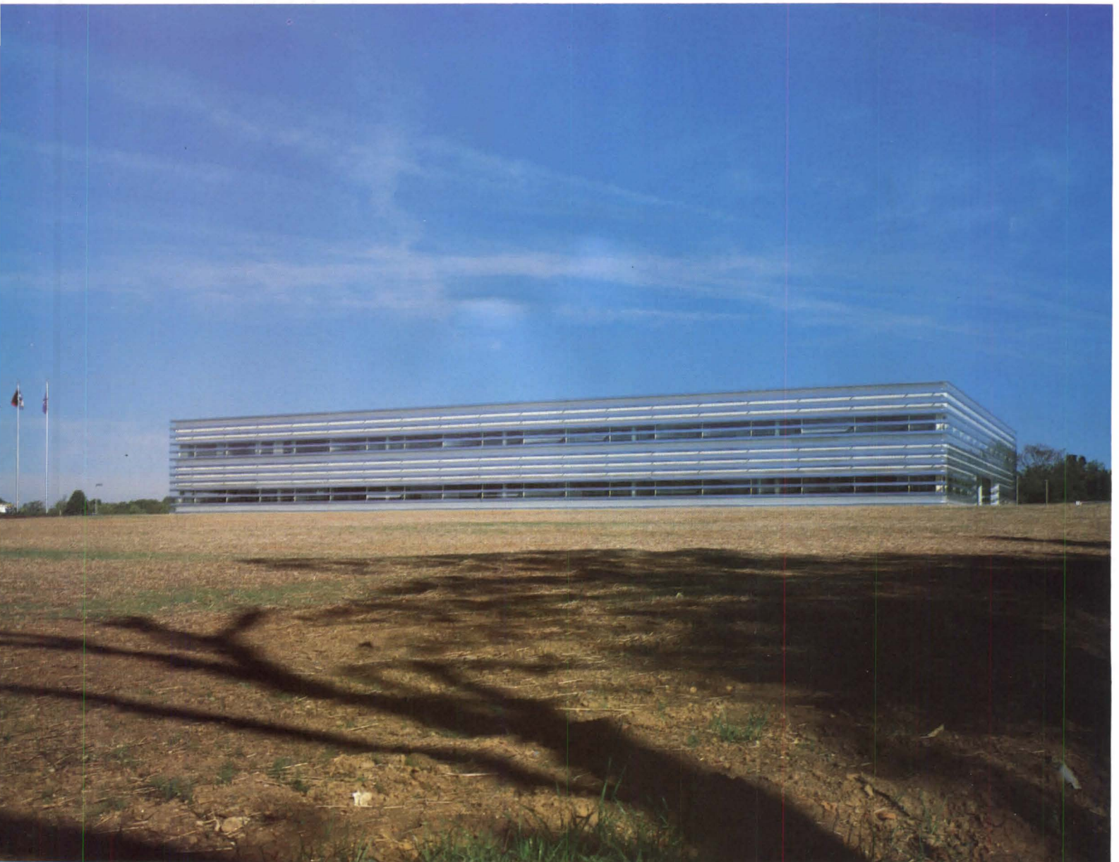
Sun warmed air is circulated through 'solar belts' to cold winter side of building.
