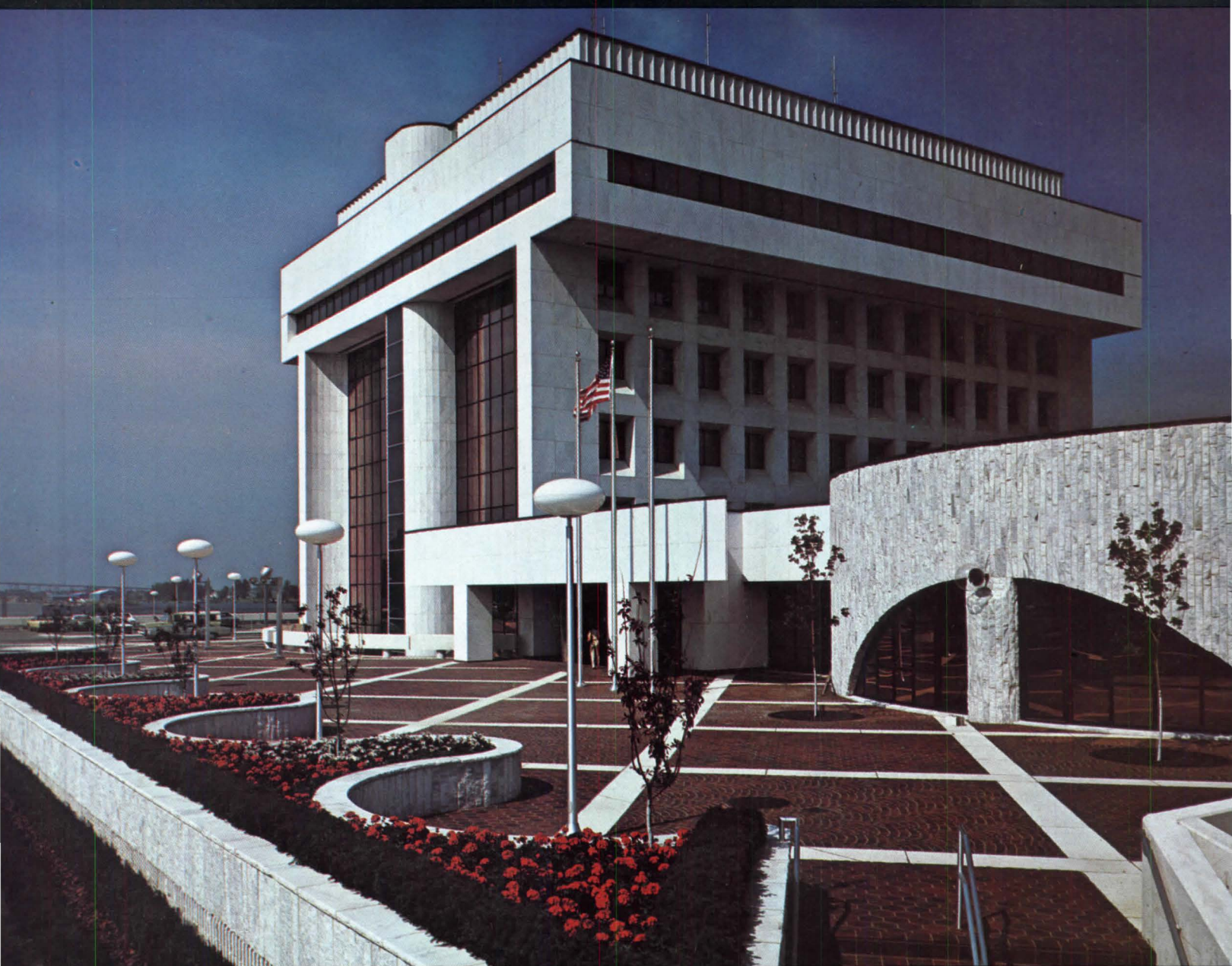
Port Huron Municipal Office Center Building, Port Huron, Michigan / All white material is Cherokee Marble / Arch: Richard C. Cogley / Marble supplied by Genesee Cut Stone & Marble Co., Flint, Michigan
