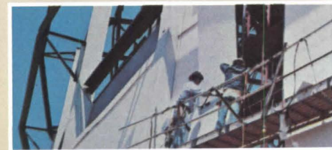
The J-M panels were face mounted to steel studding, requiring about 25 per cent less installation time than conventional masonry wall techniques.
