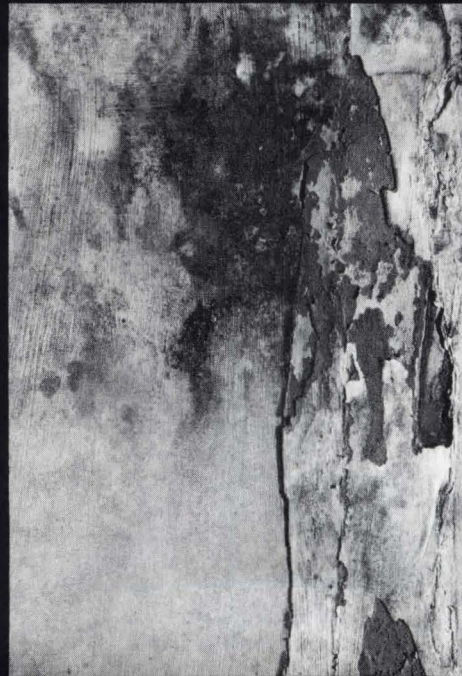
This unretouched photo shows the results of water getting behind the joint sealant.
