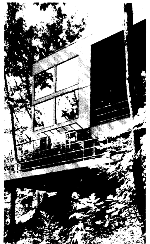
Residence on a ravine site, Chicago, northern suburb; Michael Gelick Associates, Inc., Chicago (right). The building, oriented with a north/south axis, is set deep into the site to retain existing woods and maintain privacy and provide optimum views of the ravine to the south and west from the principal living spaces. The solution is a three level building block, 32 feet wide and 72 feet long, organized with two adjacent 15-foot bays.
