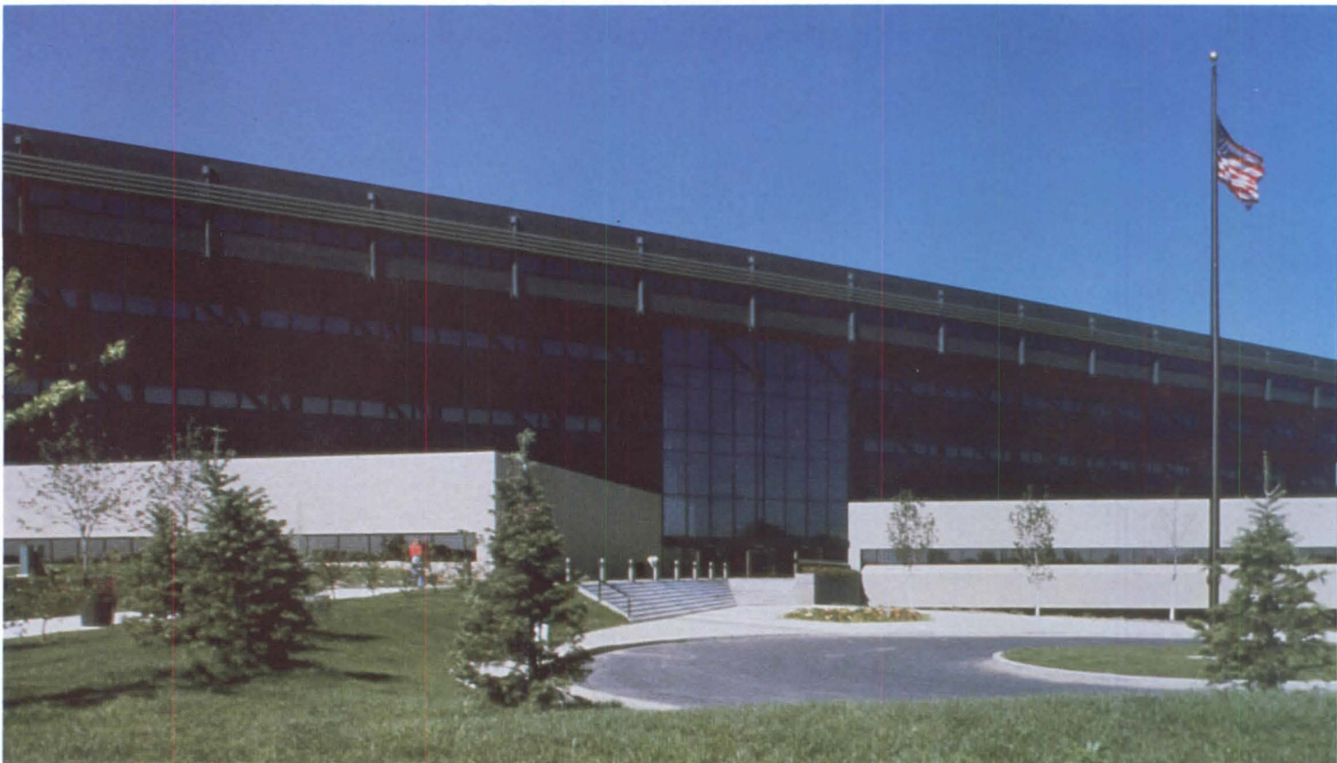
Windows on the northwest facade (left) are deeply recessed; the floors on the southeast elevation (below) are cantilevered one above the other with a sun louver on the top story and the cantilevers dramatized by an exposed steel structural frame; east facade (bottom right) presents a blank profile; atrium is shown in section, bottom left, and across page.
