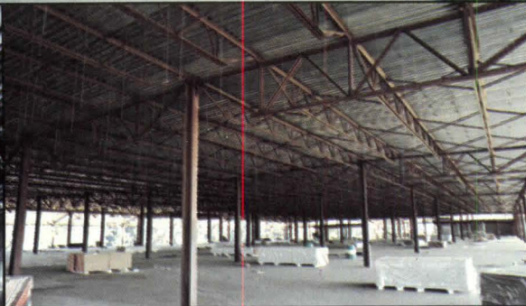
The high strength to weight of steel joists and joist girders can provide increased clear span areas, because supporting columns can be spaced further apart.
